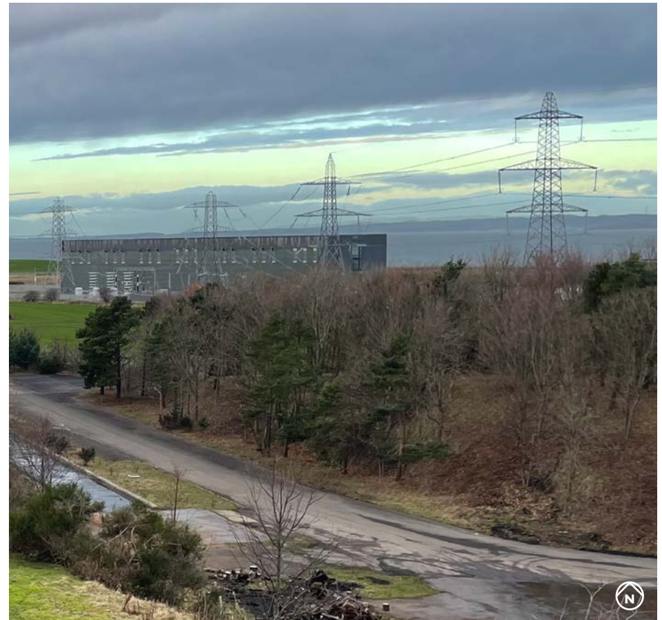
Figure 13- Existing Pylons on site
