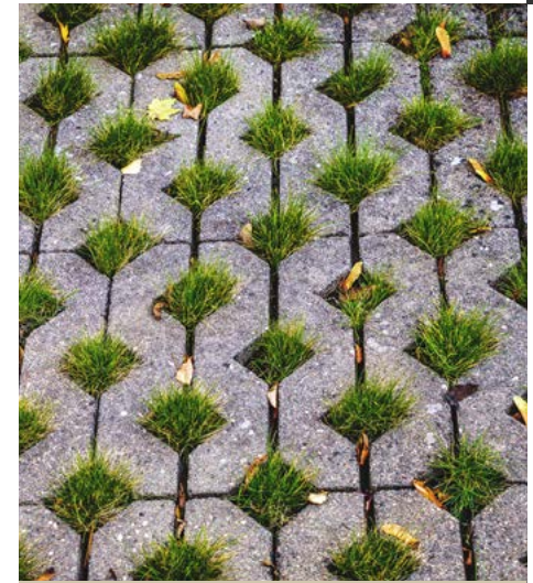
Paving which aids drainage and provides a more green aesthetic
