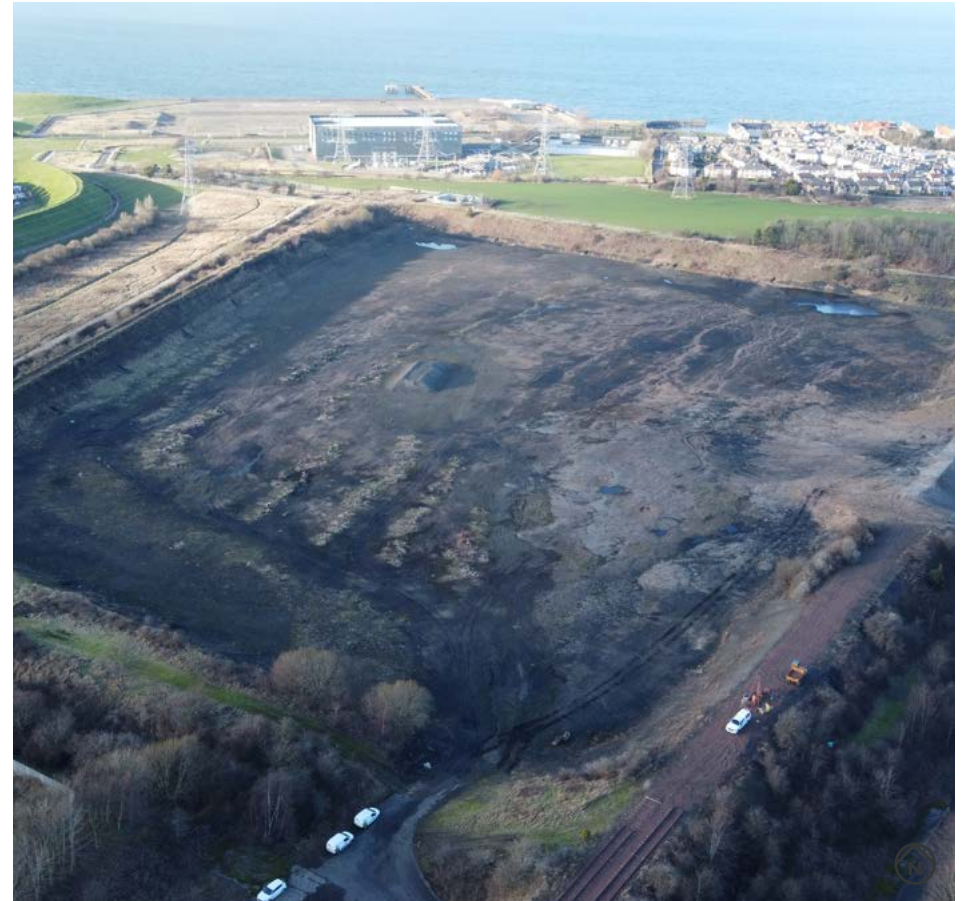
Figure 3- Coal Store Pre SLR Works
