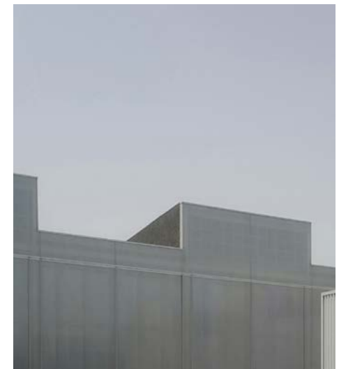
Variation in massing to break up the overall scale and differentiate between uses within the building
