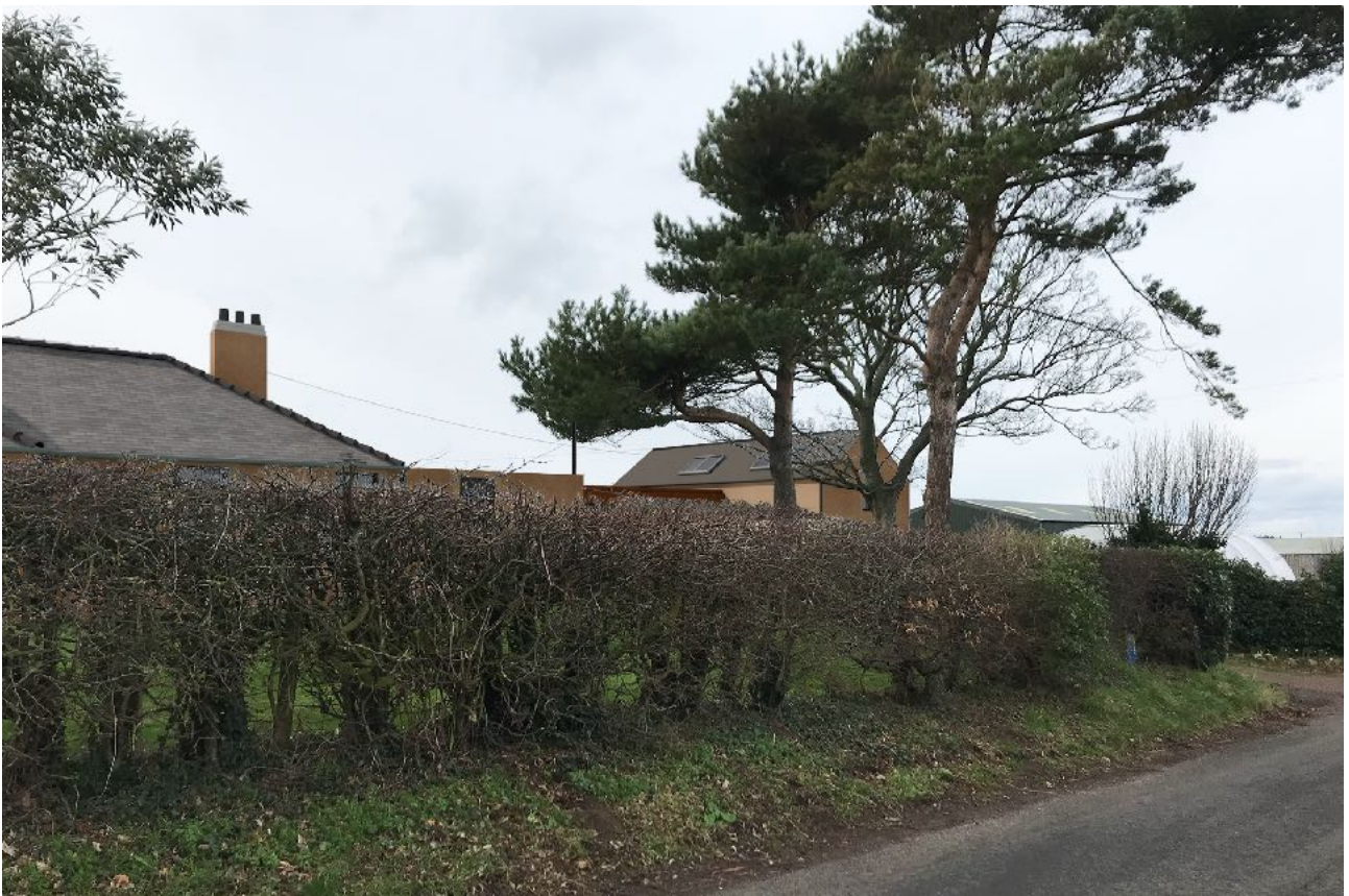
Figure 6 - Proposed photomontage. The raised height and finish of the outbuilding is most prominent. The small area of rendered extension reads as part of the house massing. The main expressed flat-roofed extension is well set back and barely visible.
