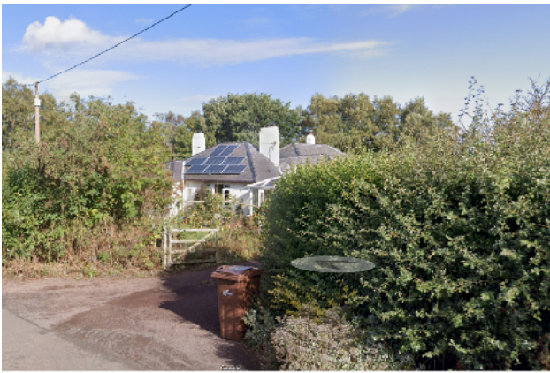
Figure 21 - 4 Newmains Holdings, significant rear extensions
