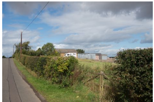
Figure 14 - Looking towards 6 Newmains Holdings
