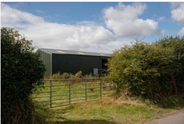
Figure 13 - Building north of 8 Newmains Holdings.
