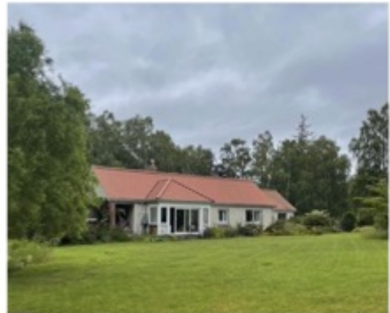
Fig. 16 Main House with Cottage behind, viewed from south-west
