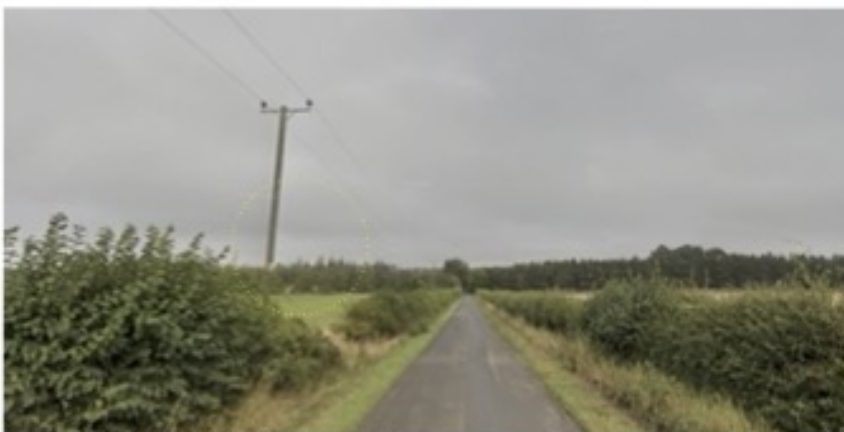
Fig. 3 View of Southwood from B1407 (indicated in yellow)
