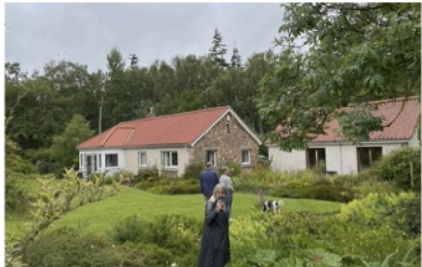
Fig. 18 The two dwellings, showing the stone gable to the eastern end of the Main House and timber windows of the Cottage
