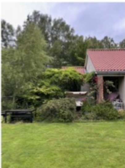
Fig. 19 Red-brick supporting pier
