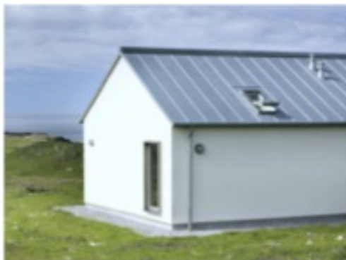
Fig 23 Rendered walls with zinc roof and rainwater goods
