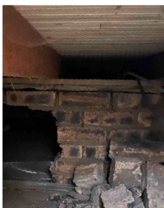
Fig. 1 Uninsulated soffit
