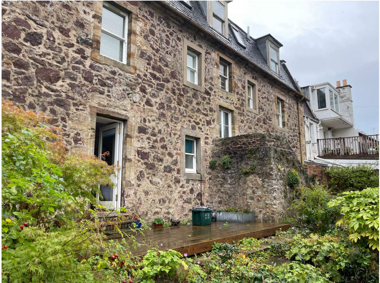
Photo 2 – see the access to the garden for Flat 2 via the bedroom door onto the decking.
