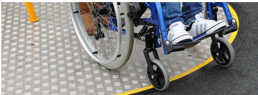
Image 10: Example of a flush transition from https://hags.co.uk/en-gb/designing-inclusive-playgrounds/accessibility
