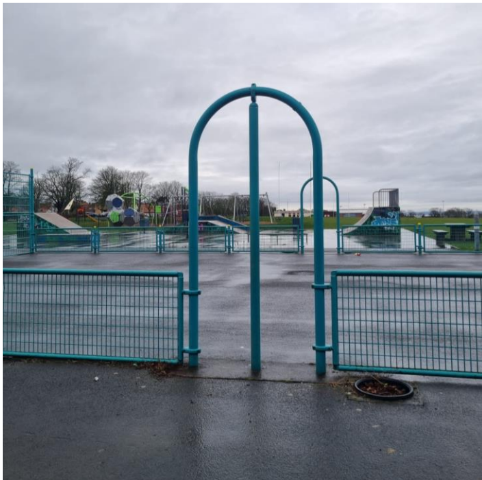
Image 5: Vertical bar blocking access to MUGA
