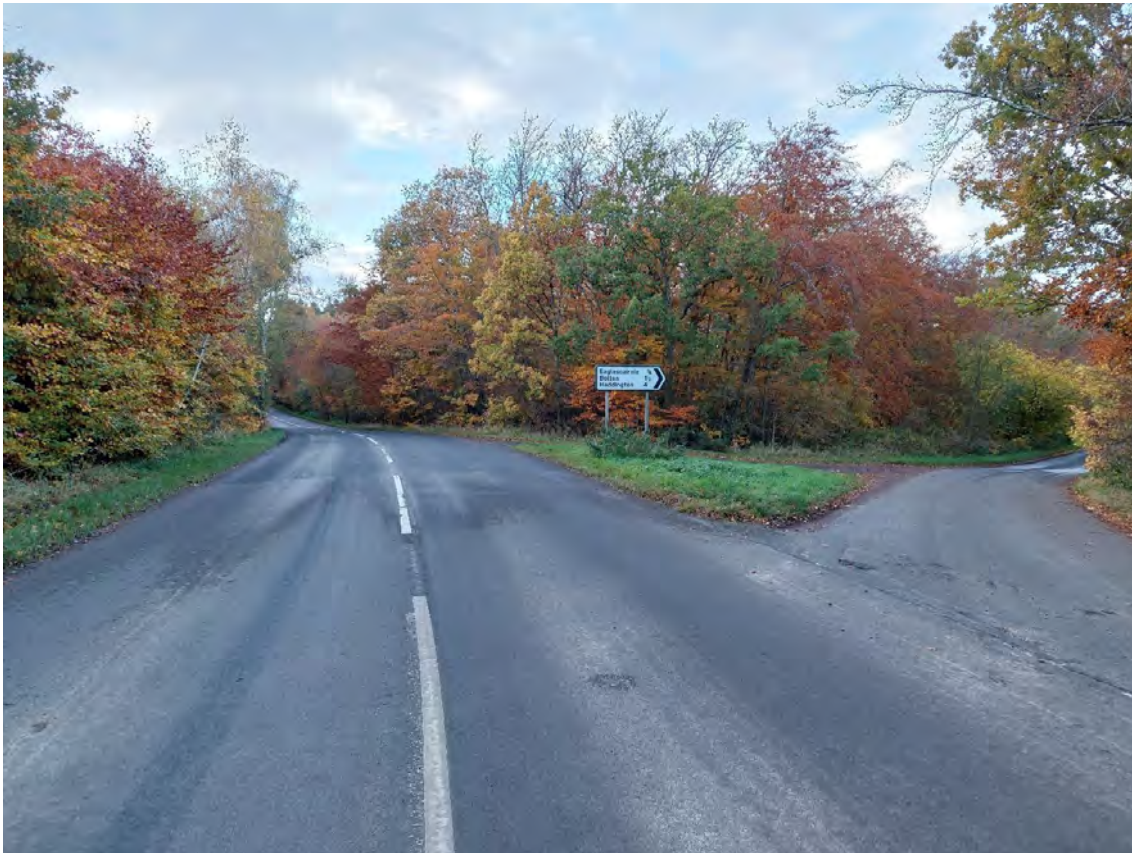
Figure 3.2 – Junction of B6355 and Unnamed and Unclassified Road
