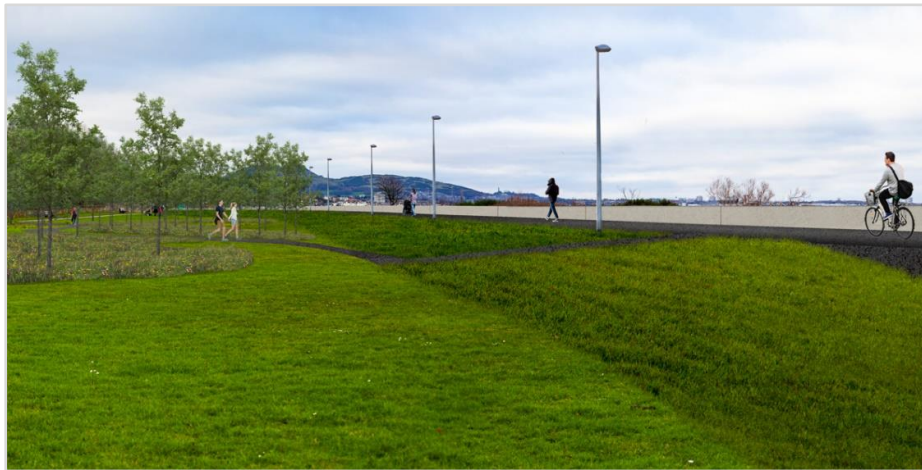
Photo 10: Hybrid embankment with short wall at Fisherrow Links
