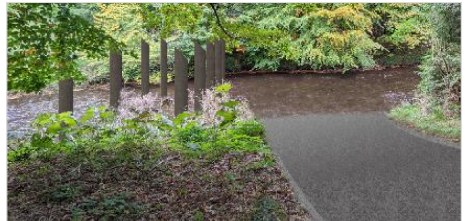
Photo 5: Photomontage of the debris trap located upstream of the A1 road bridge
