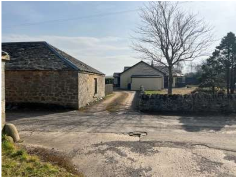
Figure 2. clash between traditional hipped roof of existing B Listed steading and gables of non-traditional 1970's bungalow
