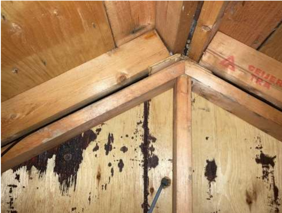
Packers used to overcome tolerance issues
