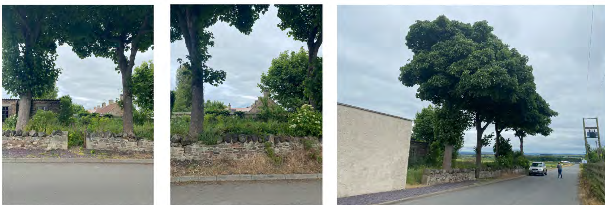
07. PHOTOS OF WALL AS EXISTING
