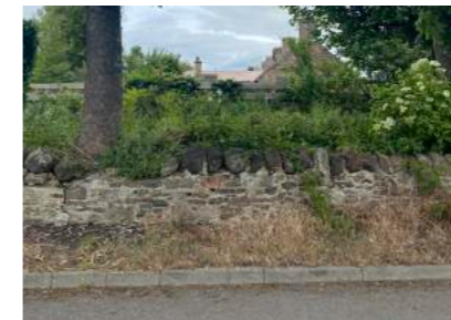
Existing Site Boundary Wall
