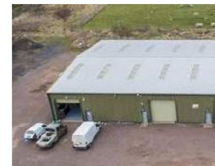
Storage Unit Sheds
