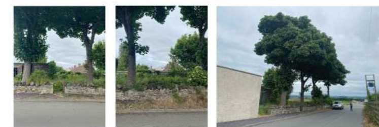
07 PHOTOS OF WALL AS EXISTING
