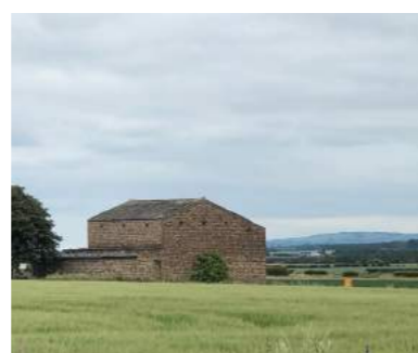
The Stand-by Set house, an auxiliary power station, still remains in good condition today
