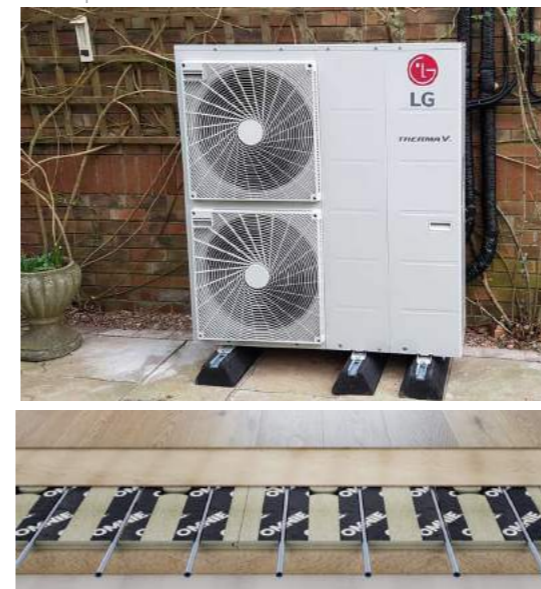
Air Source Heat Pump & Underfloor Heating examples
