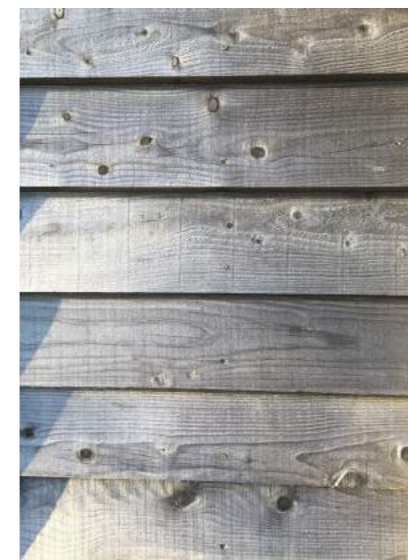
Timber feather edge weatherboarding
