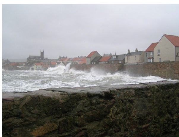
Picture 5.1: Flood damage to properties on Lammer Street, Dunbar, courtesy of Alex
