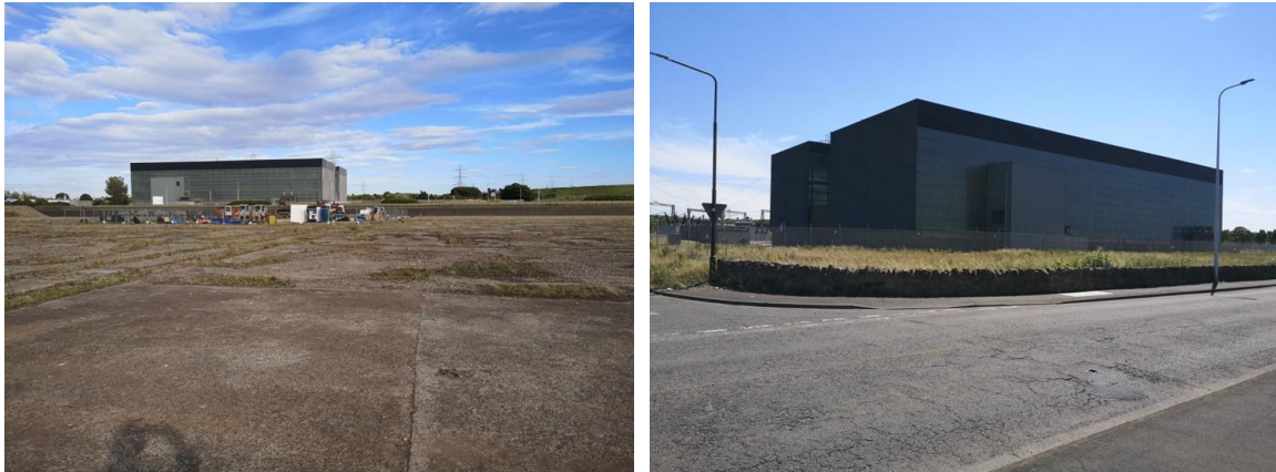
View of the existing substation from the site and roadside
