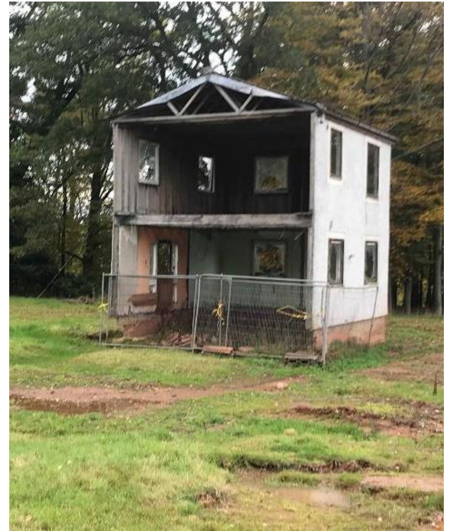
22. Close up of previous two-storey extension after demolition works,.
