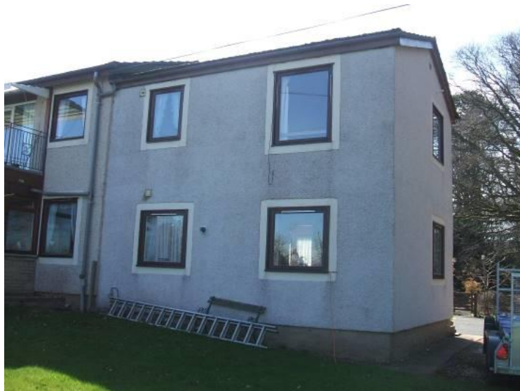
17. View from North of later two storey extension (right)
