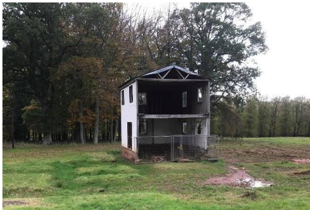
20. Remaining two-storey extensions
