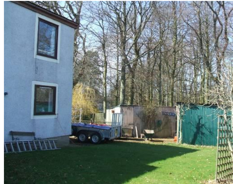
19. View from East of poor-quality outbuildings (right)
