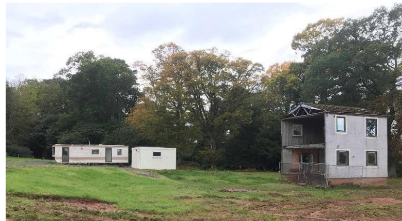
21. Two-storey extension with temporary cabin and static caravan at background
