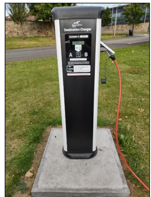
Figure 5.2 – 7-22kW Destination Charger
