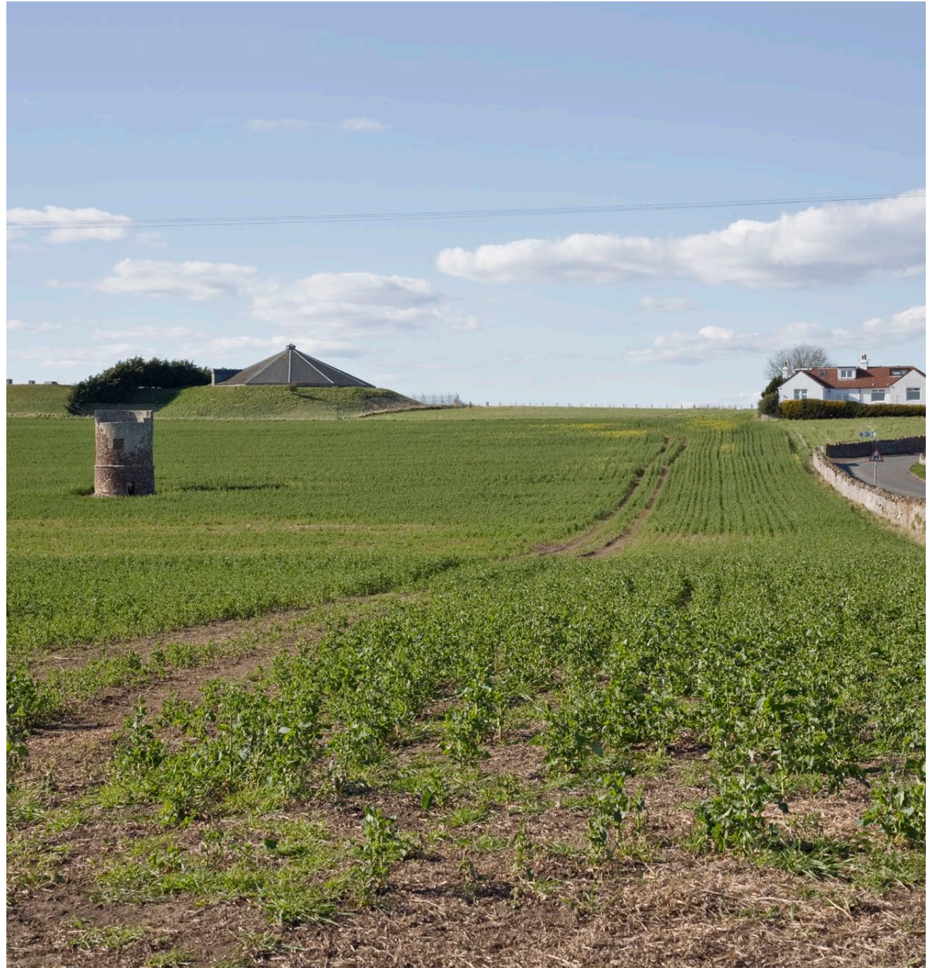
View looking north towards Dovecot, with the Water Tank and Heugh Steading in the background
