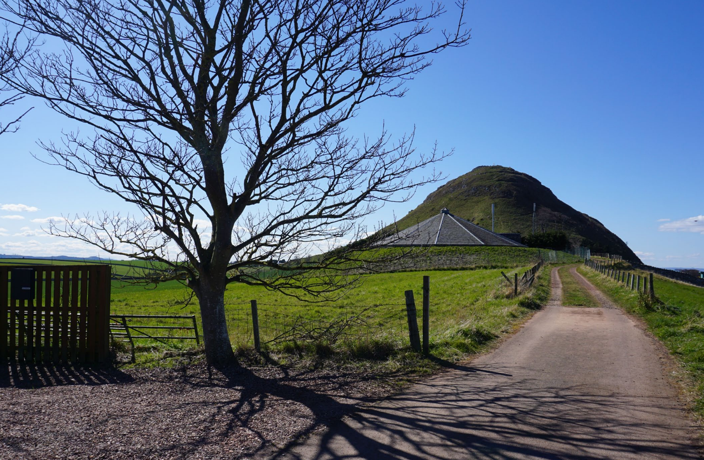
View looking west along access track with the site in the foreground and the Category B Listed Water Tower and North Berwick Law in the background
