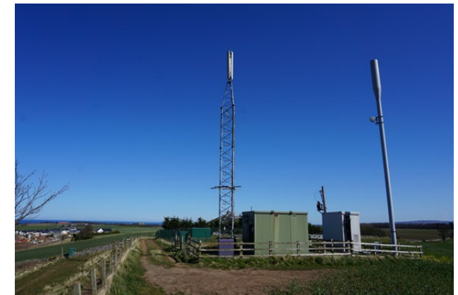
Mobile phone masts and associated infrastructure to west of Water Tower
