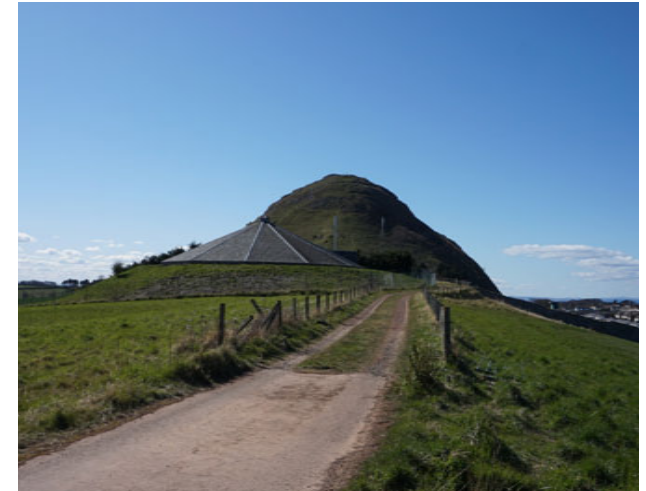
North Berwick Drinking Water Tank
