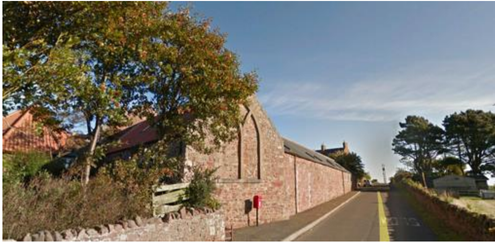
Figure 7. Heugh Steading converted to residential use, built of Law stone.
