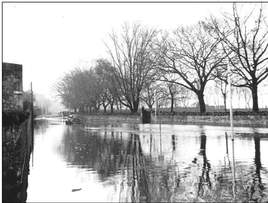
Figure 2: Flooding on New Street, looking towards Fisherrow (1948)
