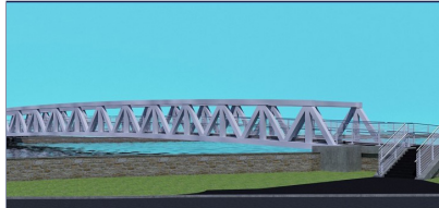
Example of a steel modified warren truss footbridge
