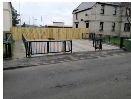
Front view of new tenants parking
