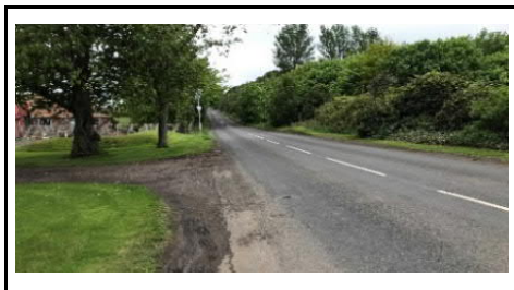
Photo 1 - A198, looking north from junction with B1407
