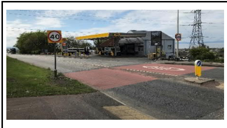
Photo 1 - A199, looking west towards 40mph terminal signs
