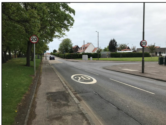
Figure 8.1 - Additional signage and painted roundel
