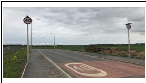
Photo 1 - B6371, looking north to 40mph terminal signs
