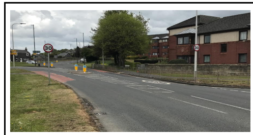
Photo 2 - Looking east towards 30mph boundary
