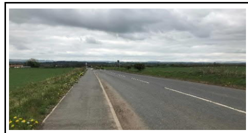
Photo 2 - B6371, looking south
