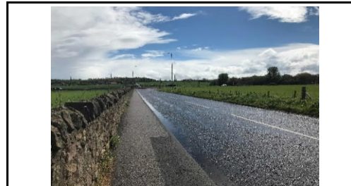
Photo 2 - A6124, looking south to terminal signs
