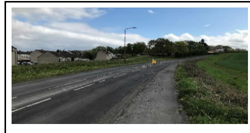
Photo 2 - B6414, looking south
