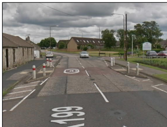
Figure 8.6 - Gateway features (e.g. build outs)
