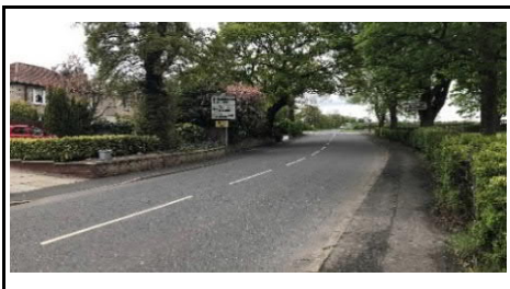
Photo 1 - Looking north-west towards terminal signs (Ref: 5202)
