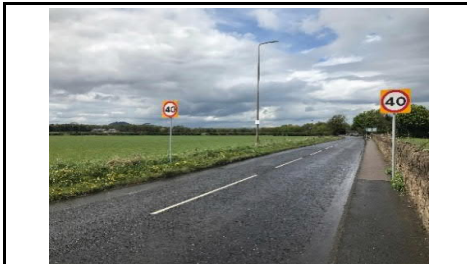
Photo 1 - A6124, looking north to terminal signs
