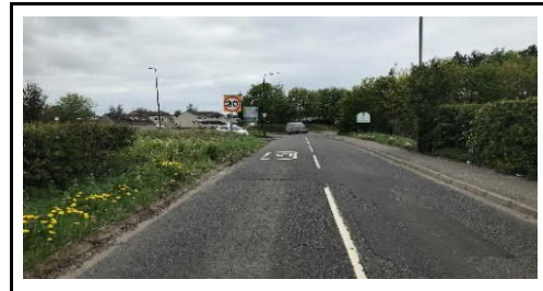
Photo 2 - B6355, looking west
