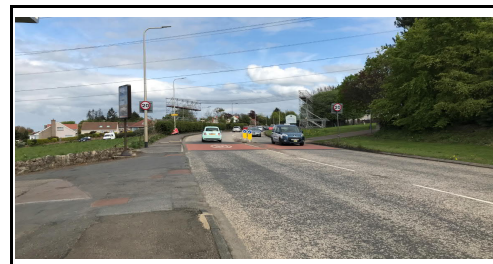
Photo 2 - Looking east towards 20mph boundary
