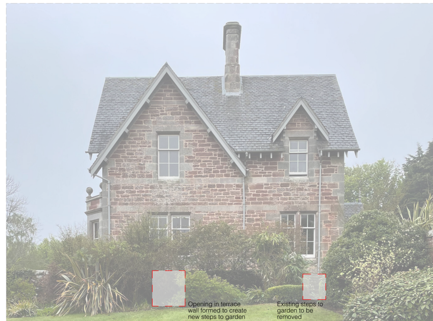
Demolition Photograph - not to scale
