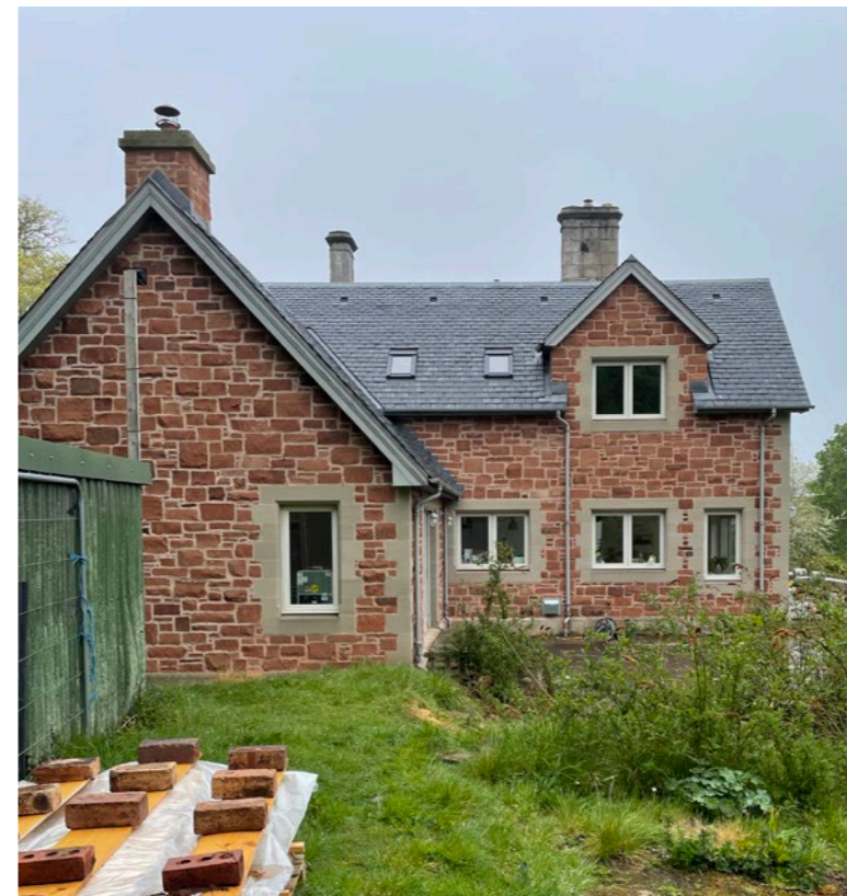
D - West frontage - modern extension
