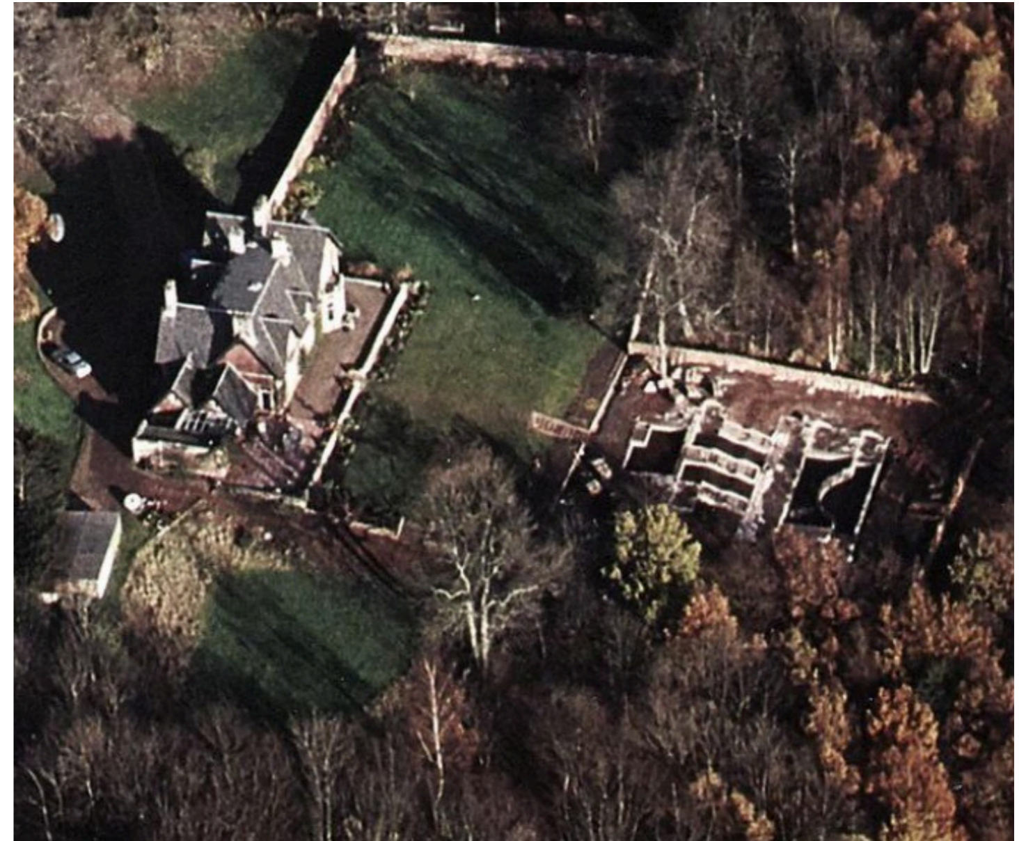
Aerial Photographs of Pressmennan House, walled garden, woodland garden and ponds Canmore, RCAHMS Aerial Photography, 2003
