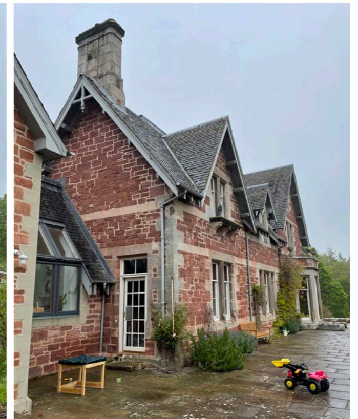
D - West frontage - original house
