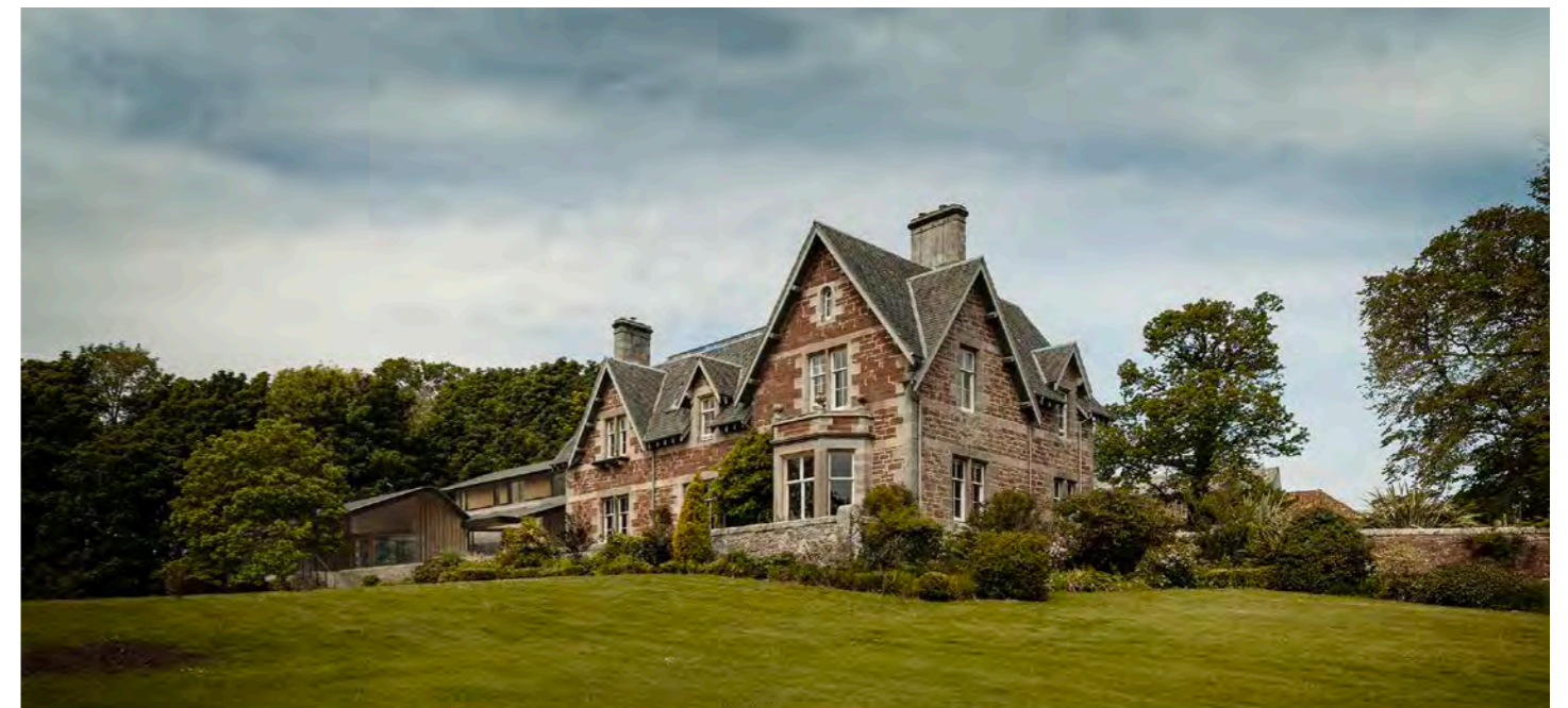
NE external view showing new proposals (top); SE external view showing view to house and proposed extension.
