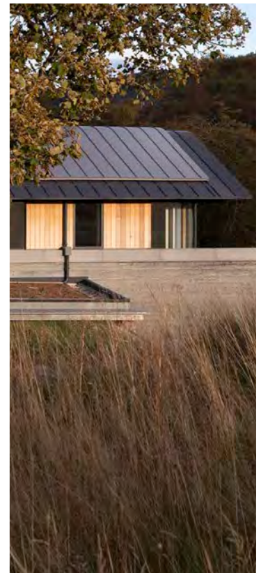
Quartz zinc roof finish on curved ridge roof
