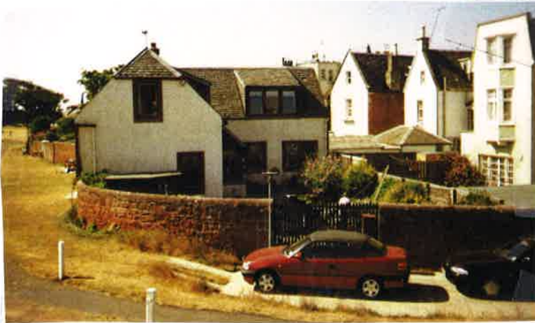
The house as built in the 1980s showing brown framed and single pane windows, completely at variance with the other properties adjoining. Taken from half way up Castle Hill.
