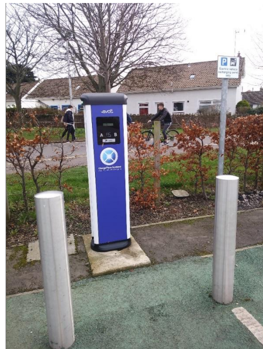
Figure 5.1 - 7-22kW AC Destination Charger
