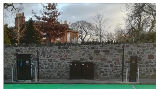
Figure 5.3 - Charging Hub in Conservation Area
