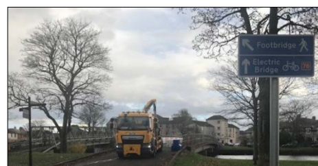
Figure 2: Installing railings and road markings prior to opening the Electric Bridge
