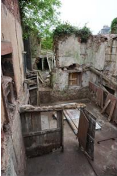
Building 4 after clearance prior to redevelopment © Addyman Archaeology
