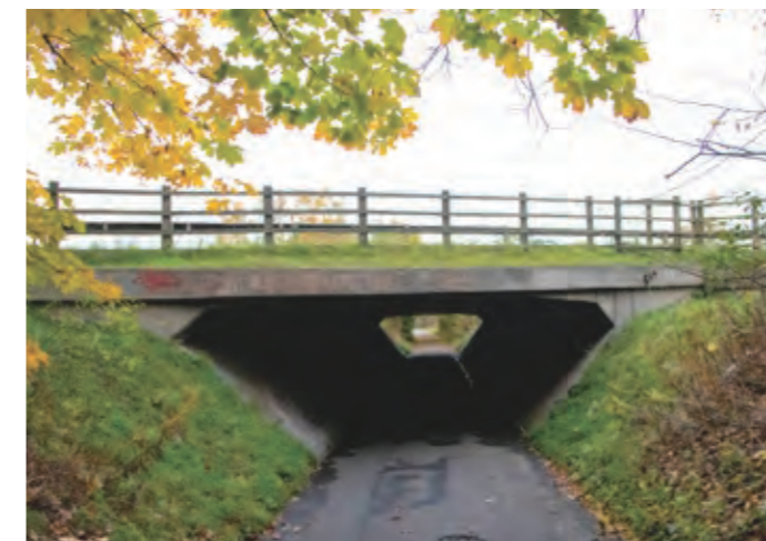
Existing underpass under the A1 north of Tranent
