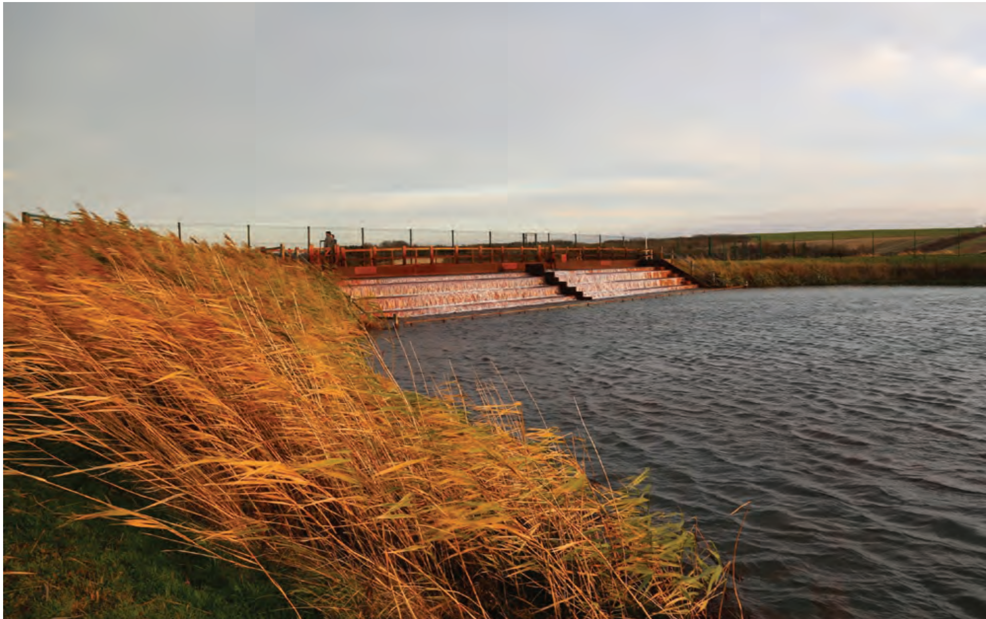
Filter ponds at Blindwells
