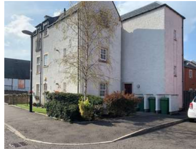
Laburnum Arch Court, Prestonpans
