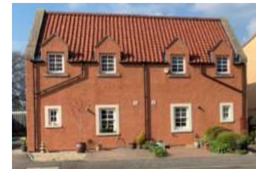
Note the use of first floor dormers that protrude above the eaves, the contrasting stone on the gable and painted outside window lining. A very effective use of detailing on a simple well proportioned house type.
