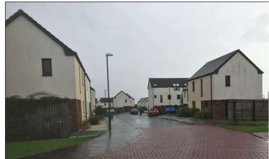
Adequate street curvature and raised table help to achieve design speed of 20mph. Source: ELC
