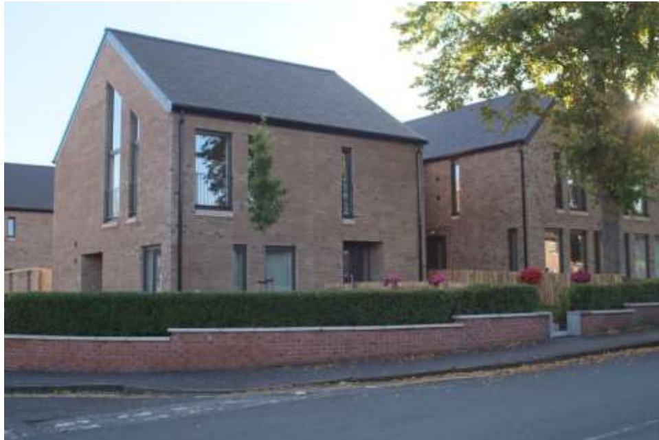
Affordable Rent Scheme at Muirsketh Rd Glasgow. Scottish Design Awards 2019 highly commended in Affordable Housing Category Credit: ELC
