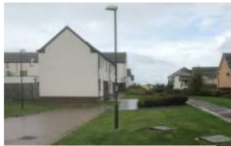
Blank gables mean occupants have maximum privacy but the street suffers as there is no natural surveillance or interesting detail.
