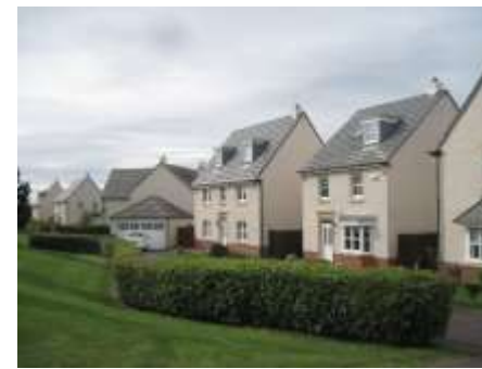
Roof mounted dormers help to add variety and to reduce the emphasis of vertical proportions on high pitched roofs.
