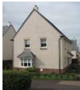
A gable with multiple windows including ground floor bay window significantly improve this house type as it adds a double front to the building.
