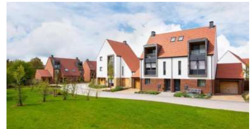
Image source: https://www.dwh.co.uk/new-homes/york/h639301-rowntree-derwenthorpe-york/
