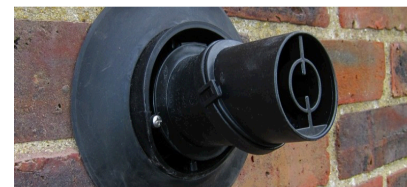
BOILER FLUE TERMINAL NTS
