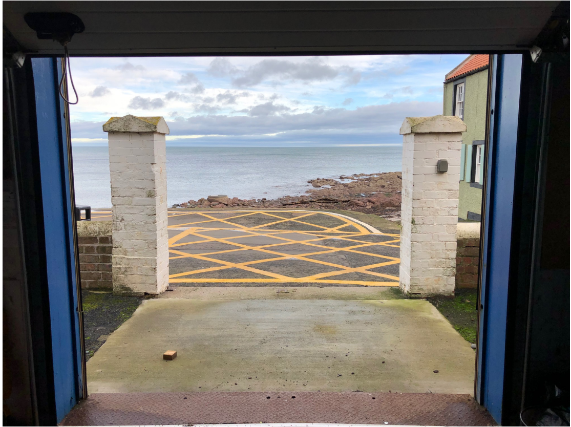
Photograph showing the view from the building and the existing vehicle access adjacent to the carriageway.
