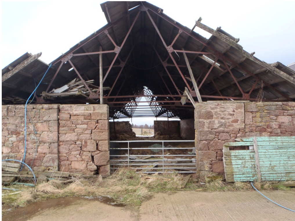
Picture 4: showing a view of building 3B
