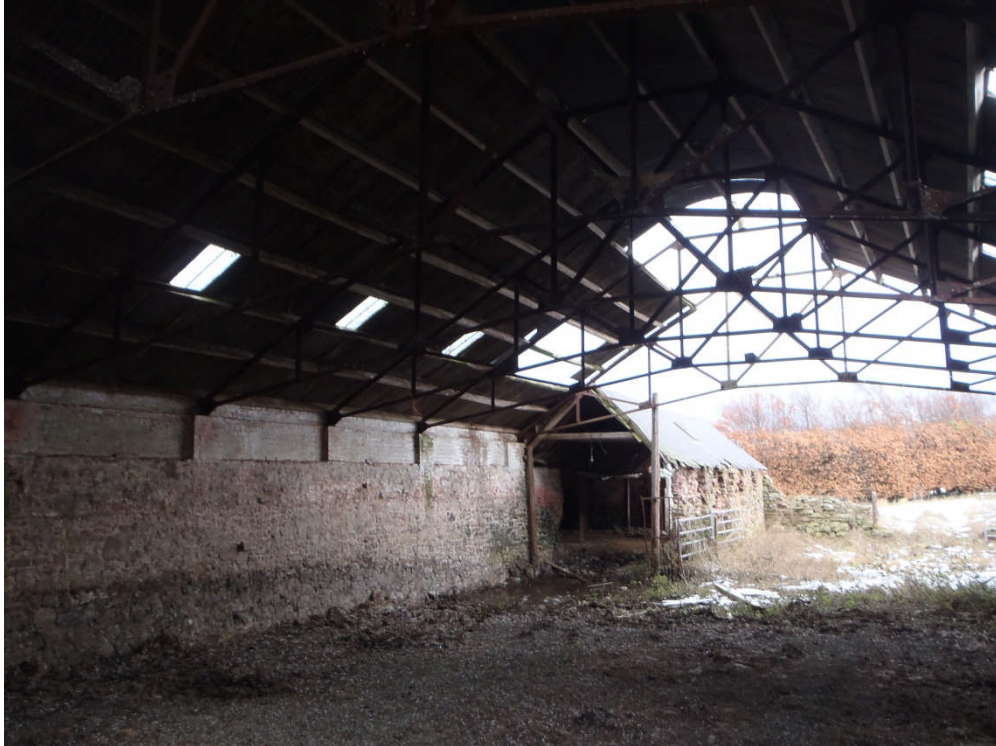
Picture 5: showing a view of building 4A and 4B
