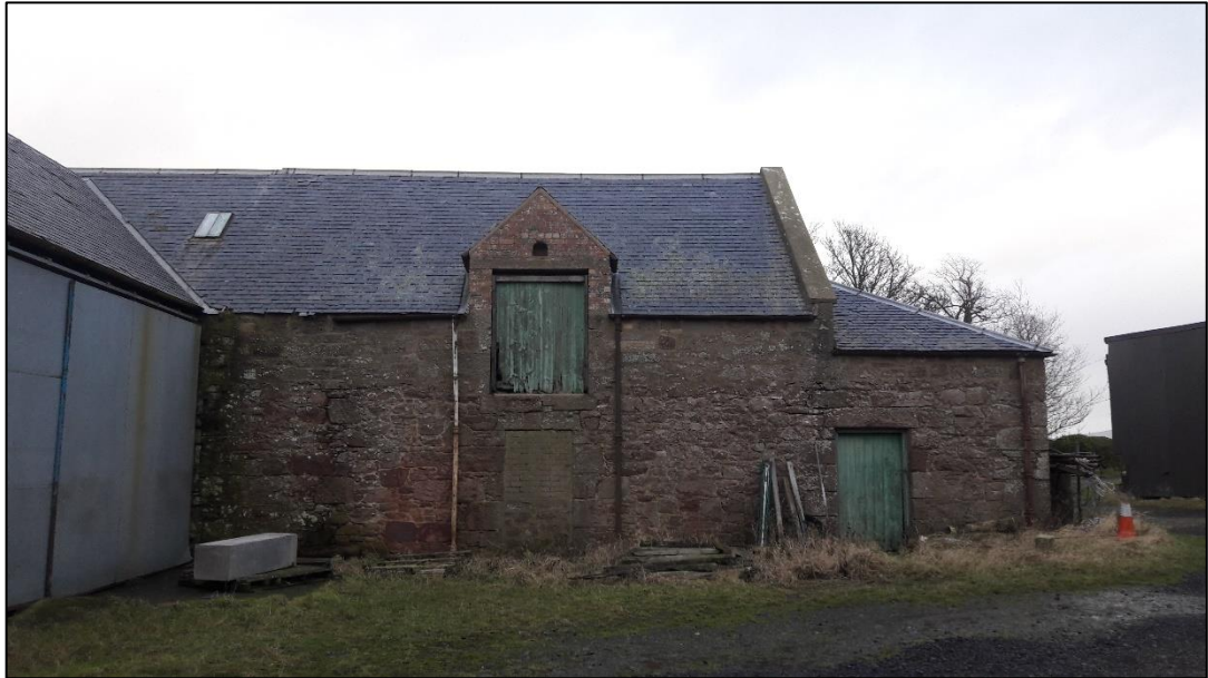
Fig 7: Attractive traditional Building - to be retained (unit 9, western elevation)
