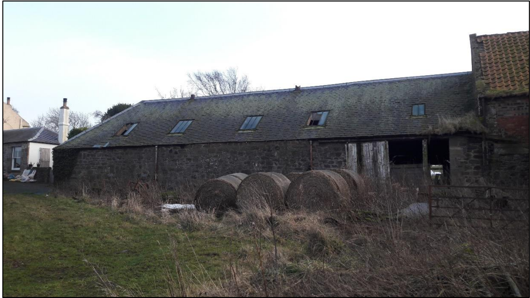
Fig 5: Traditional building (unit 7, northern elevation) – to be retained
