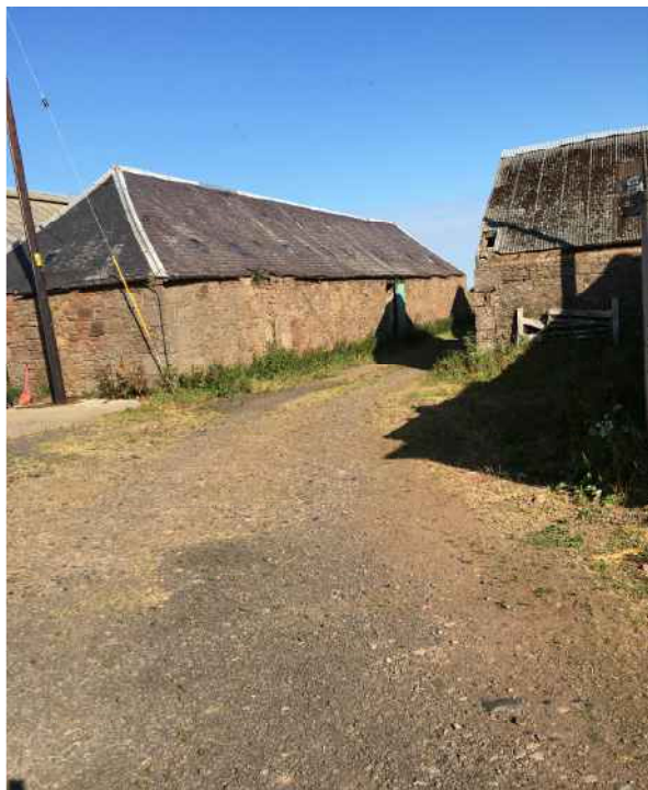
Looking north-west across central portion of site.
