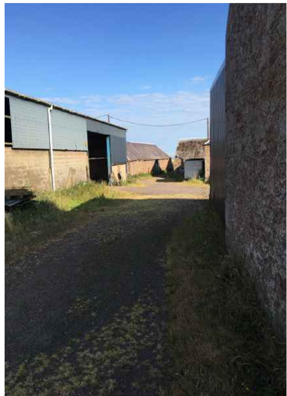
Looking northwards across sites western portion 2018
