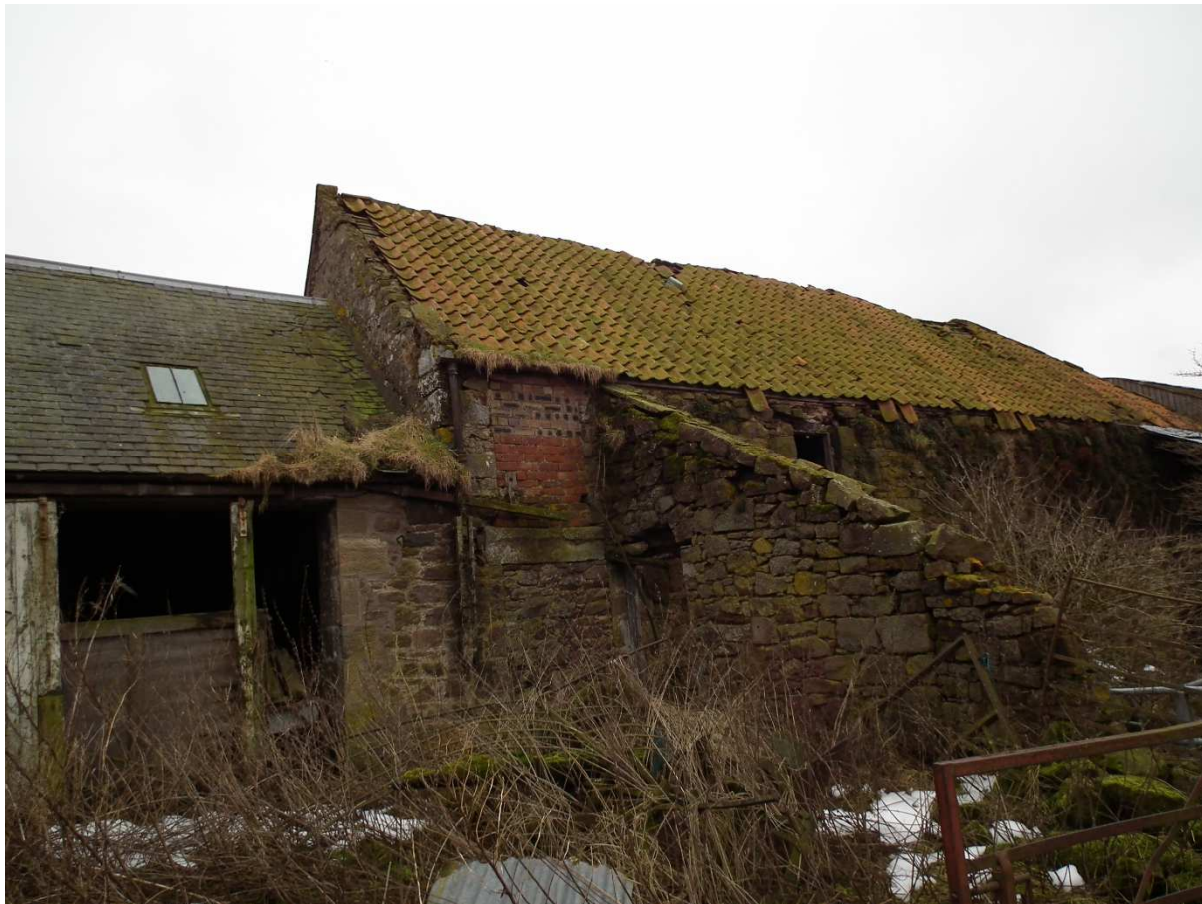
North Wall of Block D, Building G.
