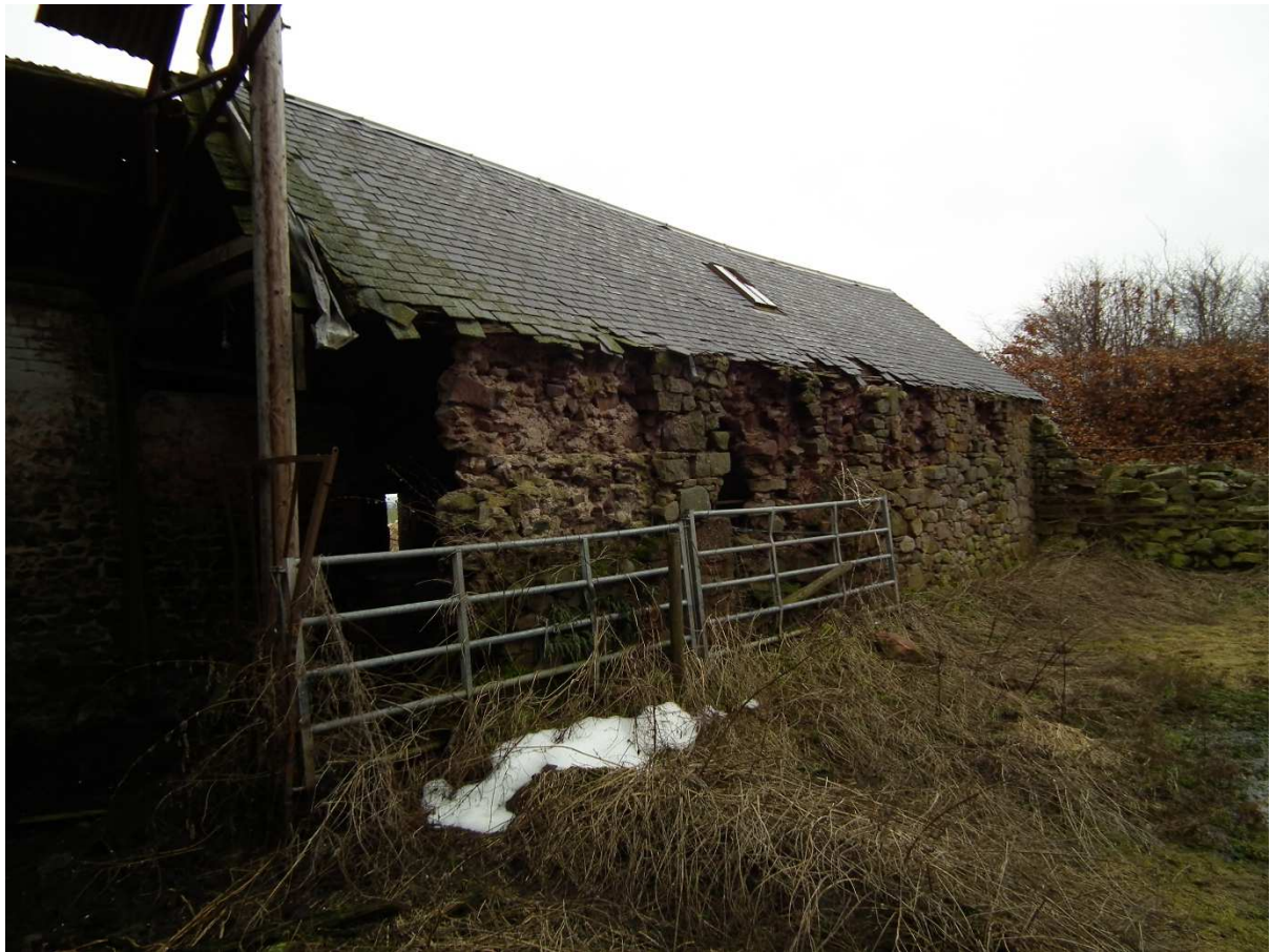
South Wall of Block E, Building H.
