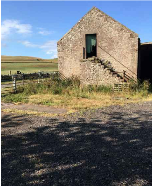
Building on southern portion to be retained
