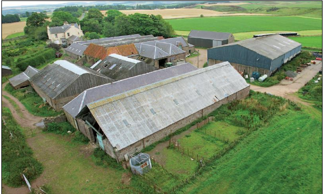
Fig 2: Overview of Longnewton Steading (view east)
