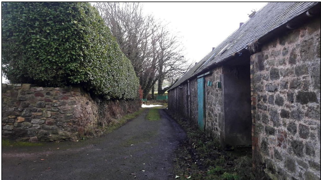
Fig 6: Traditional building (unit 7, eastern elevation) – to be retained
