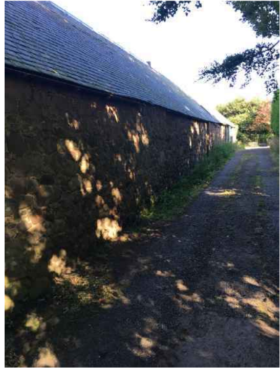
Part of building on eastern portion to be retained.
