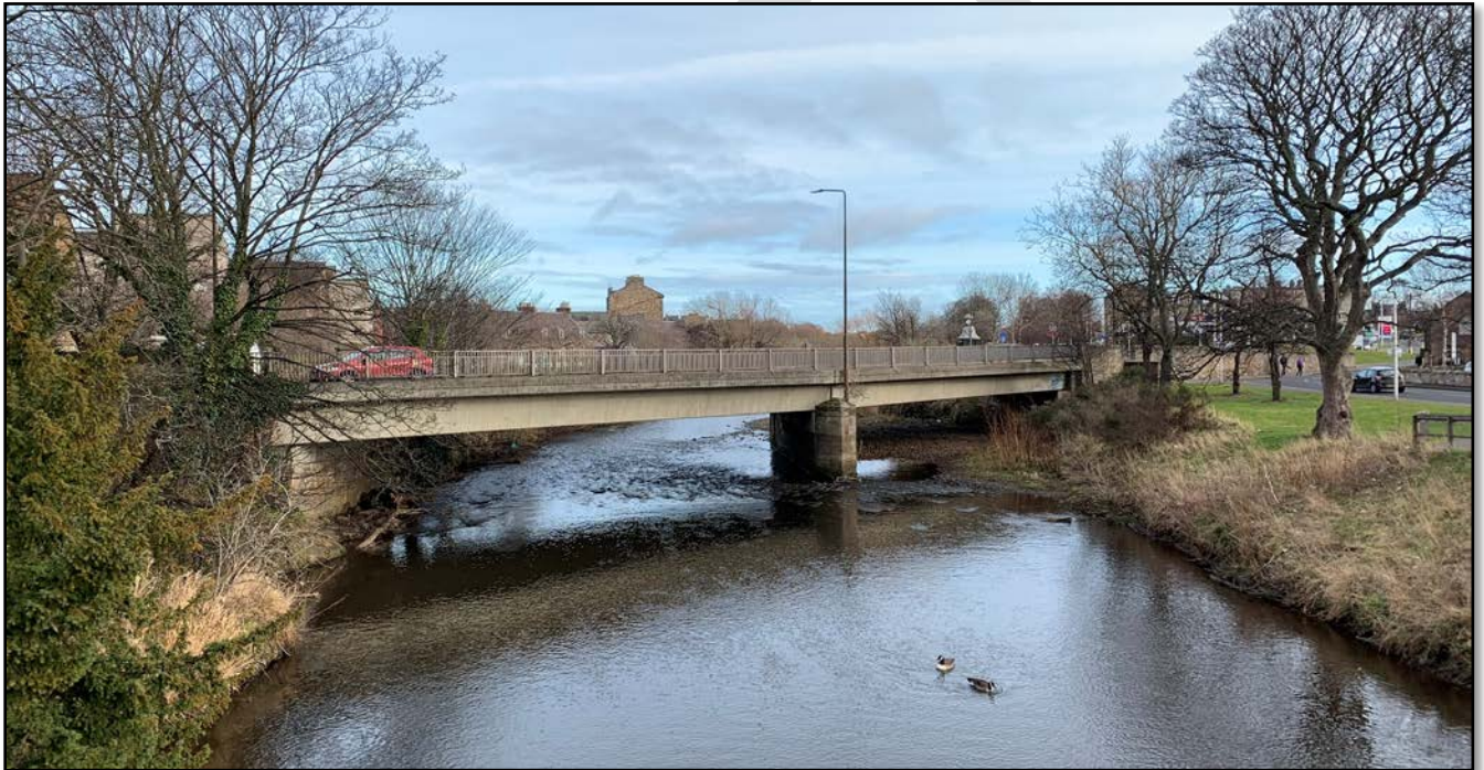
Figure 3.7: Olive Bank Road Bridge
