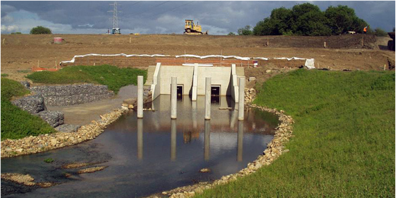
Figure 3.32 – Example of debris trap for large trees and debris at River Gaunless, County Durham
