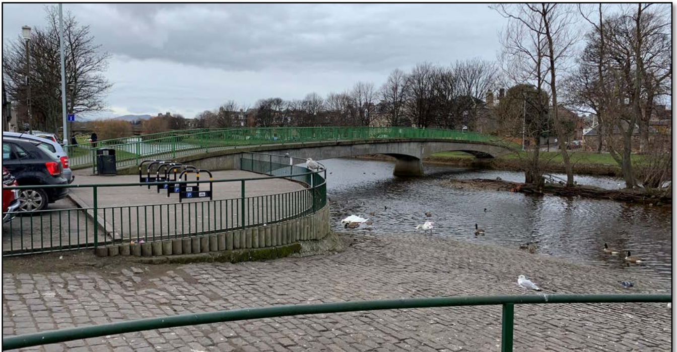
Figure 3.14: Shorthope Street Footbridge
