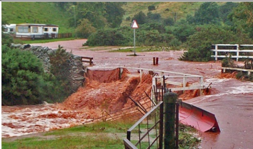
Figure 18: Flooded road in the Lammermuir Hills near Oldhamstocks
