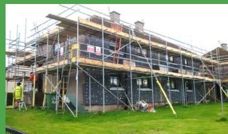
External wall insulation is installed on housing at Pinkie Braes, Musselburgh
