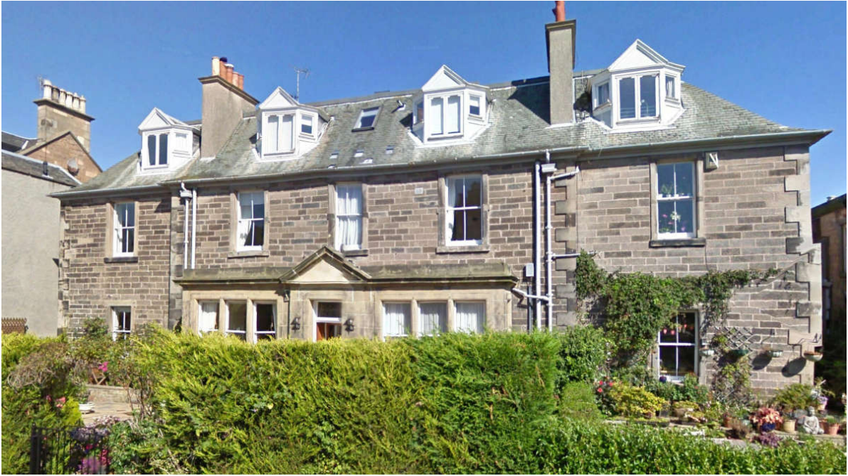
20 WEST BAY ROAD VIEWED ON GOOGLE EARTH.
