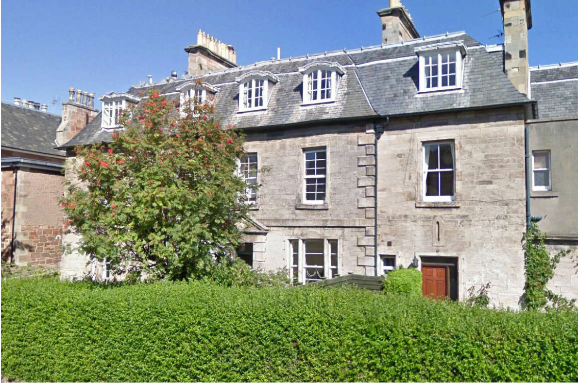
10 WEST BAY ROAD VIEWED ON GOOGLE EARTH.
