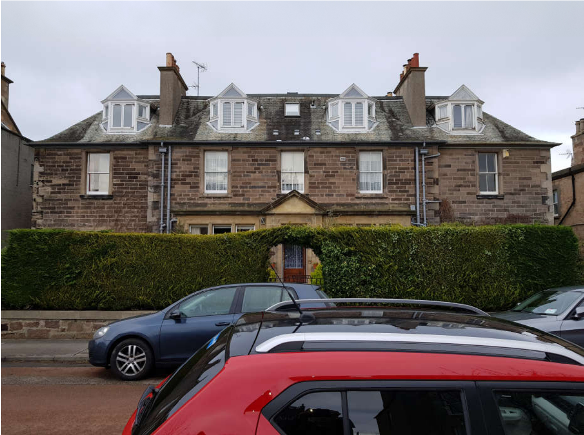
20 WEST BAY ROAD VIEWED FROM STREET LEVEL.
