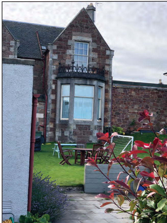
PLATE 4: No. 12 Westgate, detail of the westernmost bay of the original villa, from the NNE
