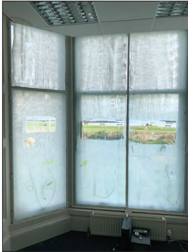
PLATE 13: Room 6, detail of the bay window from the SSE
