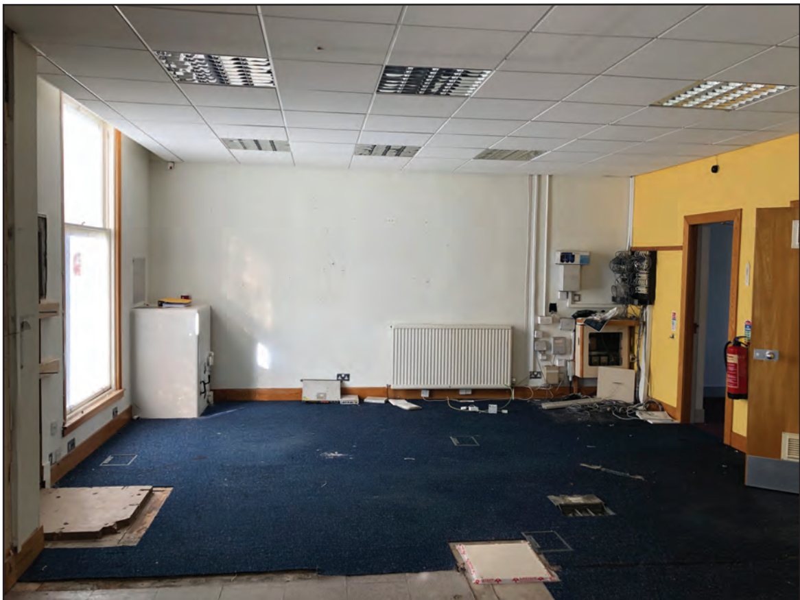
PLATE 8: Room 2, general view from the east
