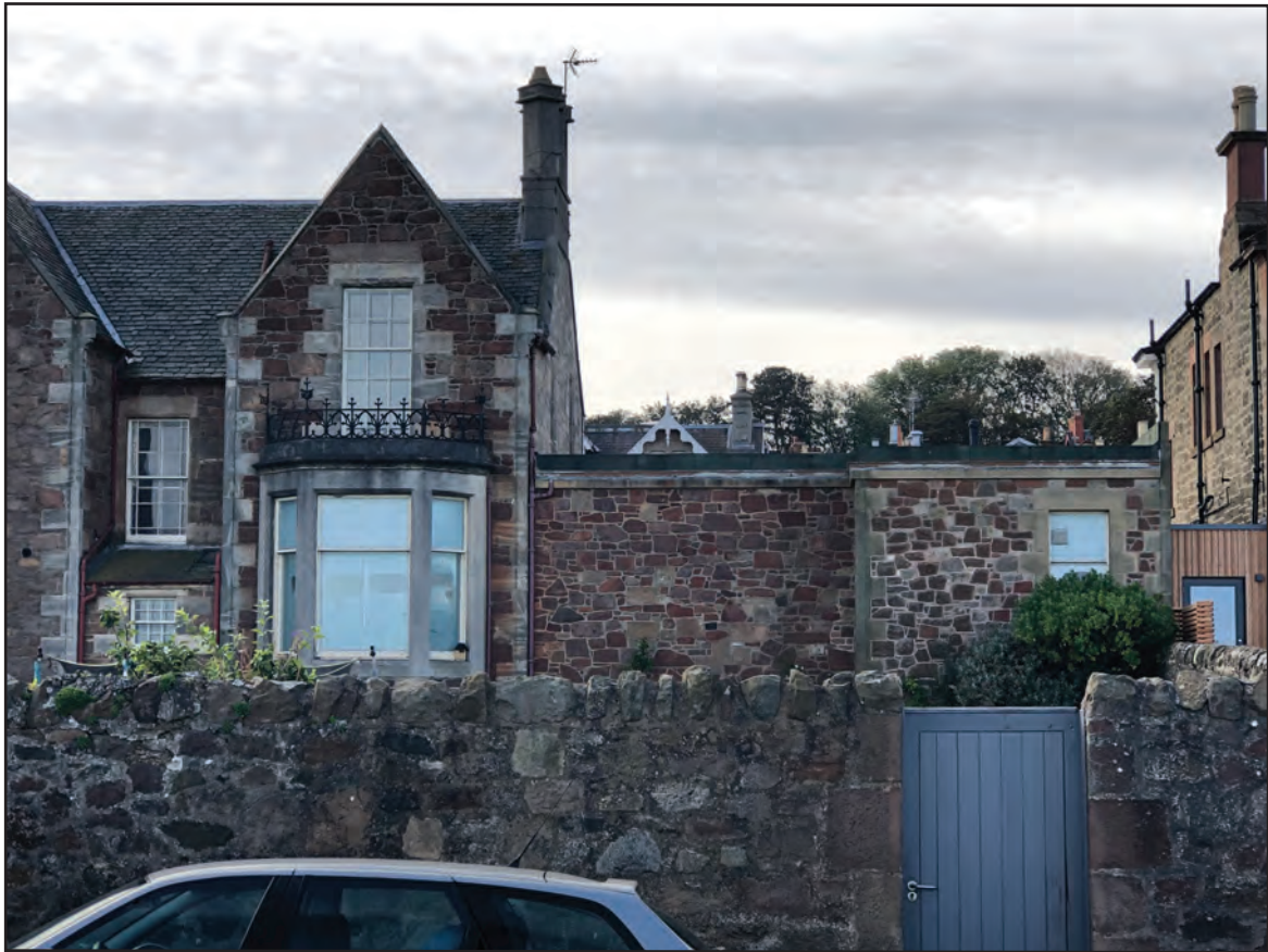
PLATE 5: No. 12 Westgate, general view with the later extension, from the north
