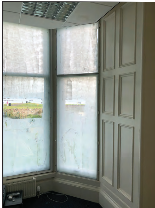
PLATE 14: Room 6, detail of the bay window from the south-west
