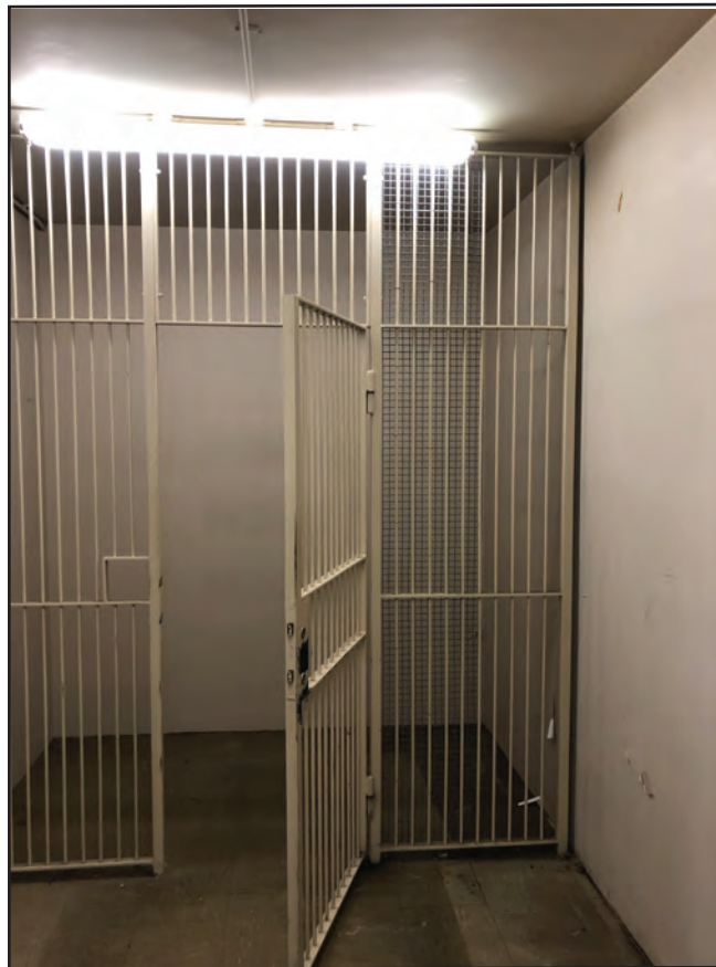
PLATE 12: Room 5, general view showing caged safe, from the east
