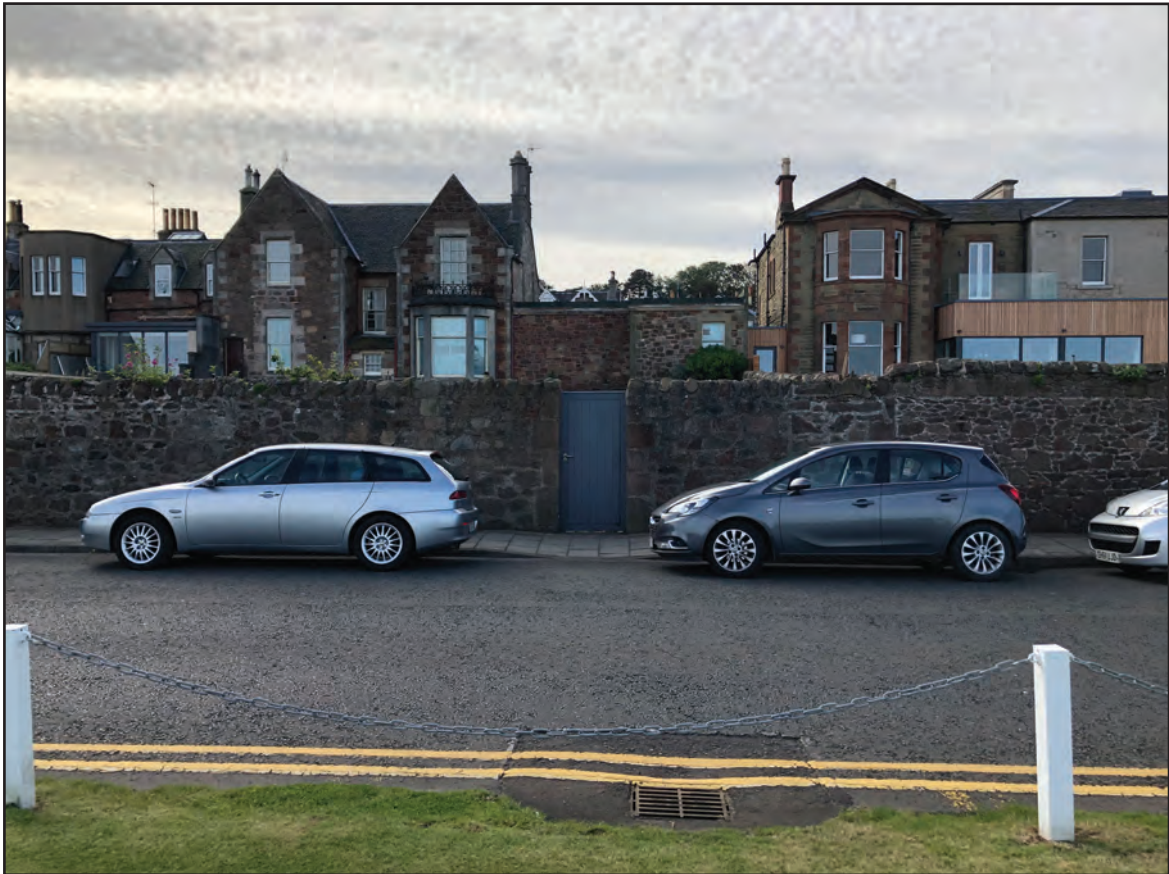
PLATE 3: No. 12 Westgate, general view of the north elevation, from the north
