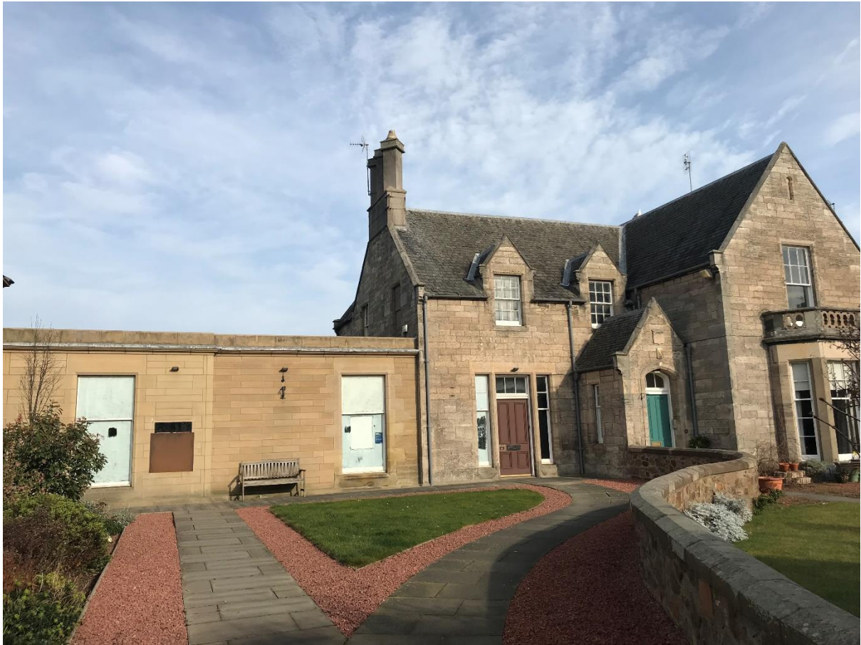
12 Westgate 'Park House', North Berwick.
