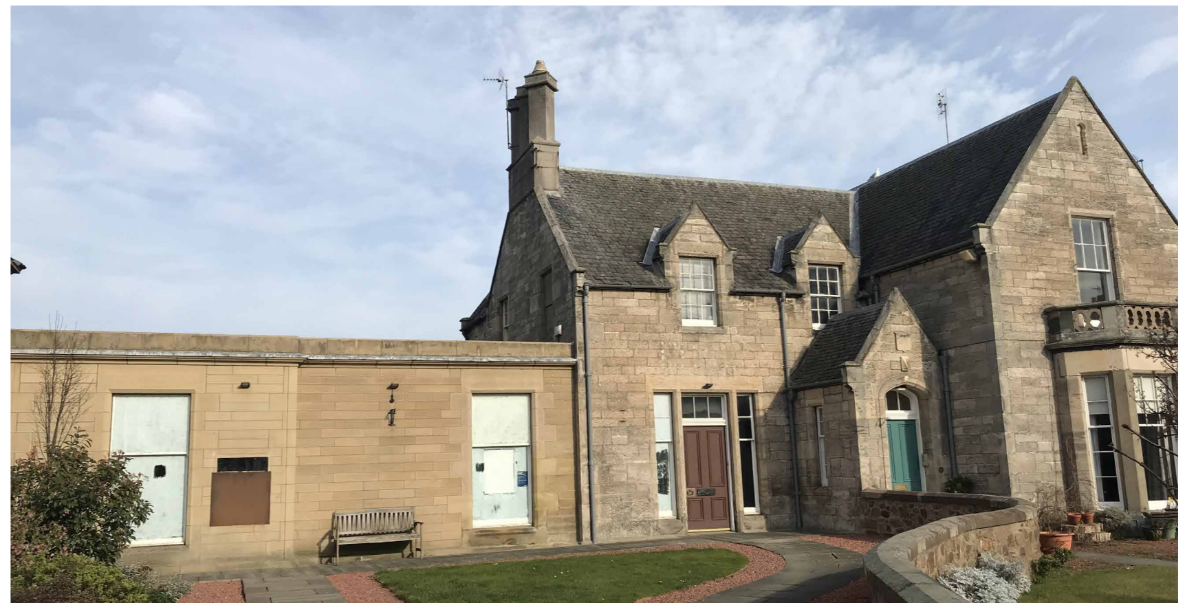
View of the property from Westgate at the site's access point
