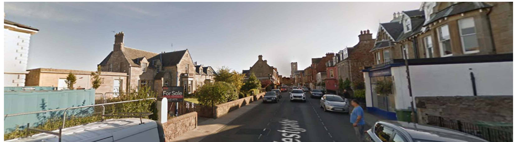
View looking East from the junction at Bank Street with the application site to the left. Again the clear definition from the residential area to the town centre can be seen here along with extensions to residential properties at ground floor level. To the right the extension is built right up to the street to reflect the pattern of the town centre. The add on of the bank building is also distinguishable although set back within the site.
