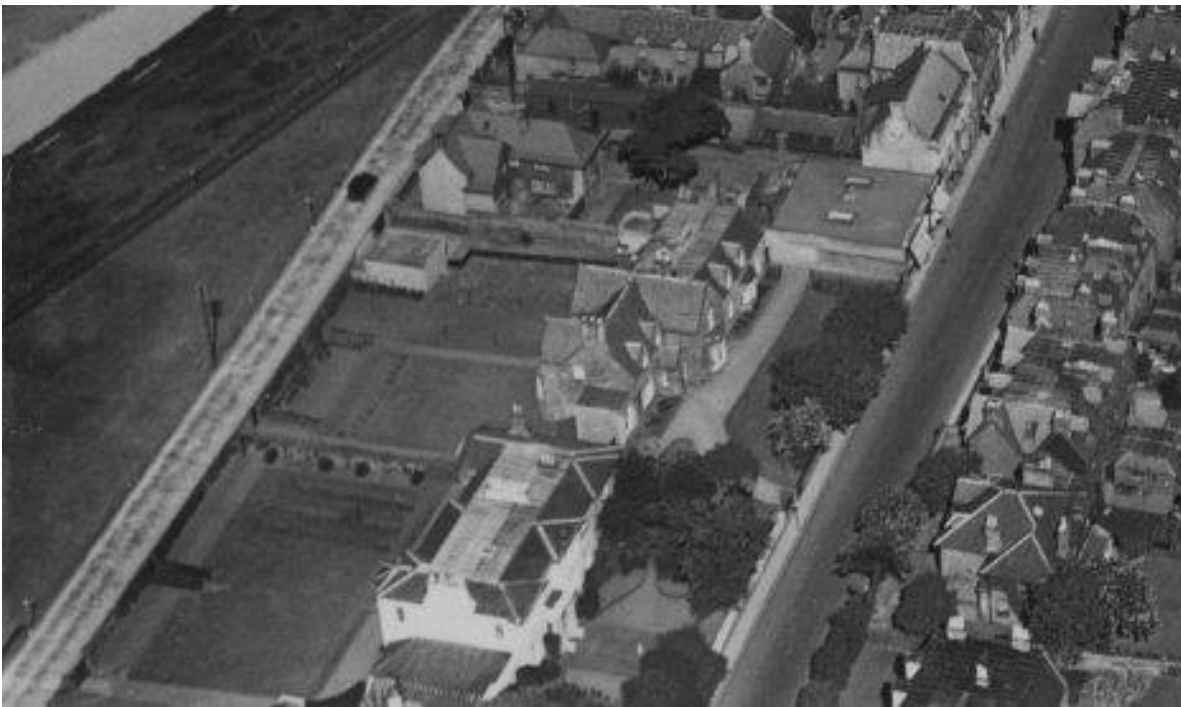
Historical aerial image showing a side extension previous to the banking hall and a driveway accessing the site.
