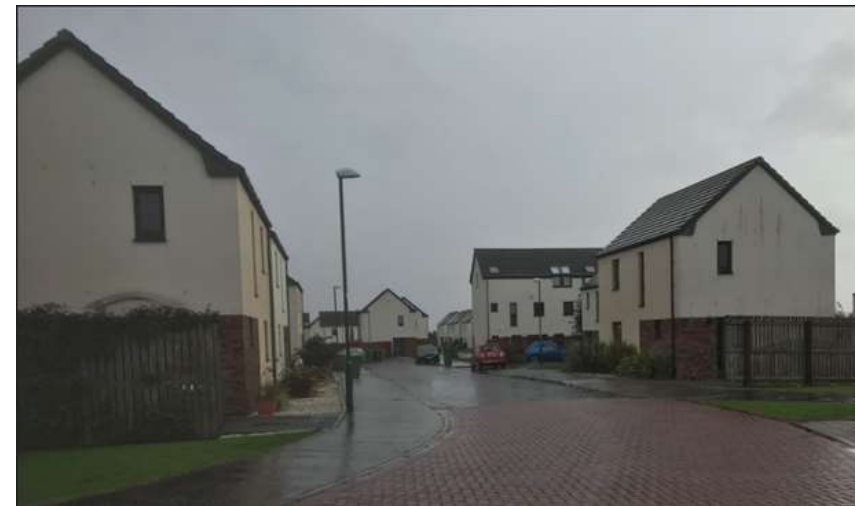
Adequate street curvature and raised table help to achieve design speed of 20mph
