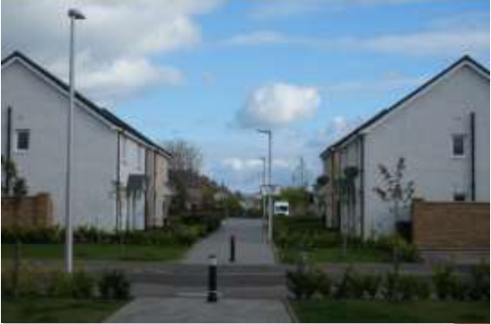
Pinkie Farm Musselburgh (first from the bottom) – pedestrian & cycling link between new development and existing street network
