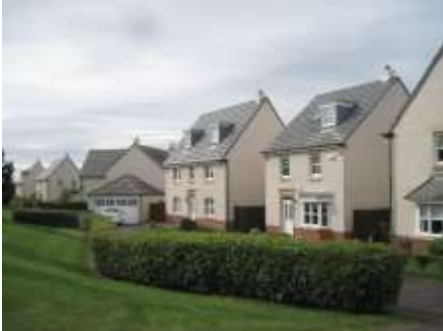
Roof mounted dormers help to add variety and to reduce the emphasis of vertical proportions on high pitched roofs.
