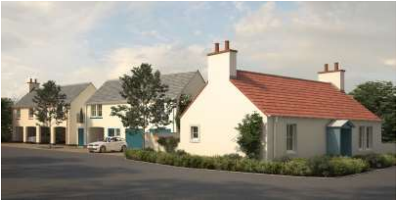
Image source: 18/01038/AMM Longniddry South Phase One, Site B - Planning & Design Statement (September 2018)
