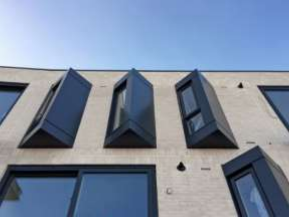
Angled oriel windows help to increase privacy. Barns Place, Oxford (RIBA South Regional Award 2017). Source: https://www.habhousing.co.uk
