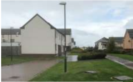
Blank gables mean occupants have maximum privacy but the street suffers as there is no natural surveillance or interesting detail.
