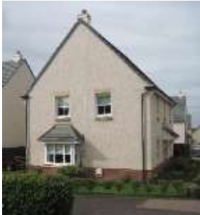
A gable with multiple windows including ground floor bay window significantly improve this house type as it adds a double front to the building.
