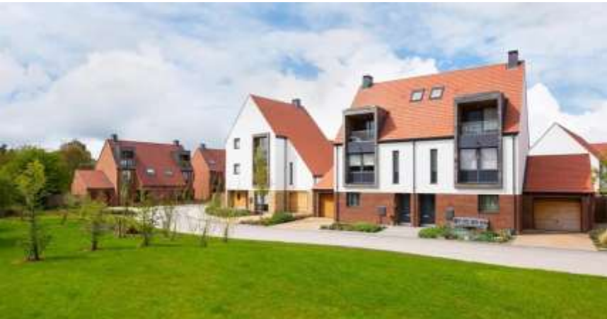
Image source: https://www.dwh.co.uk/new-homes/york/h639301-rowntree,-derwenthorpe,-york/
