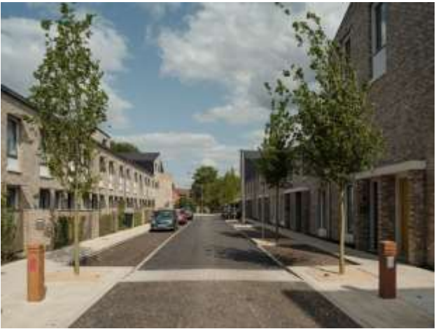
Goldsmith Street, Norwich; source: https://www.architecture.com This high-density development of council houses won the 2019 RIBA Stirling Prize Award.
