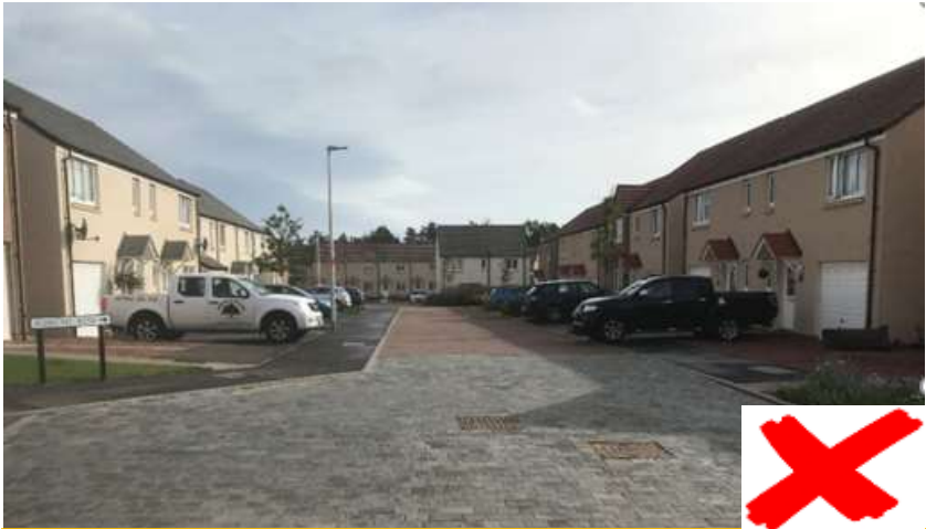
Front parking dominates the street scene. Prominent integrated garages have detrimental impact on the streetscene.
