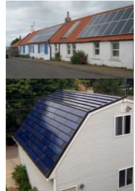
The top example shows poor integration of solar panels on a roof through the stark difference in colour. The bottom example shows much better integration of solar panels.
