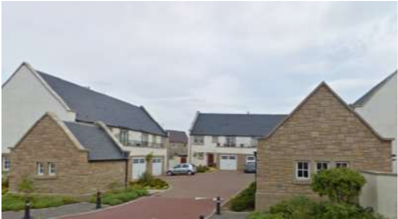
Nungate Gardens, Haddington
