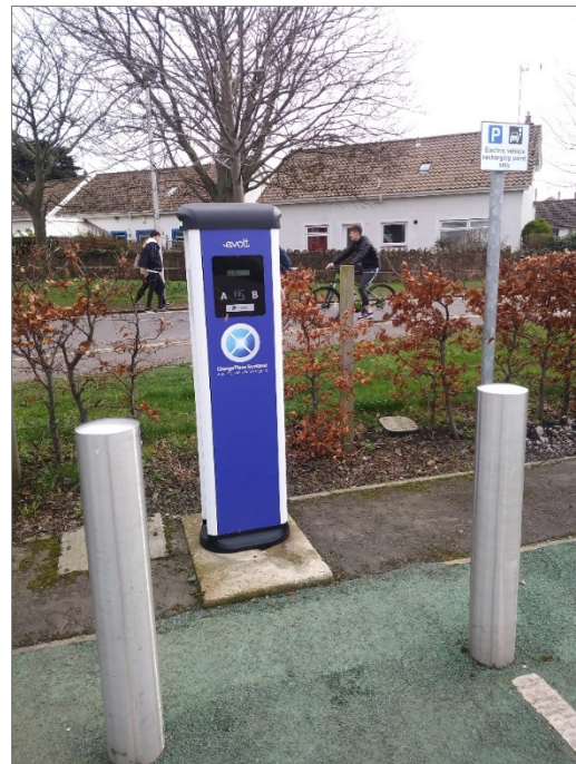
Figure 5.1 - 7-22kW AC Destination Charger
