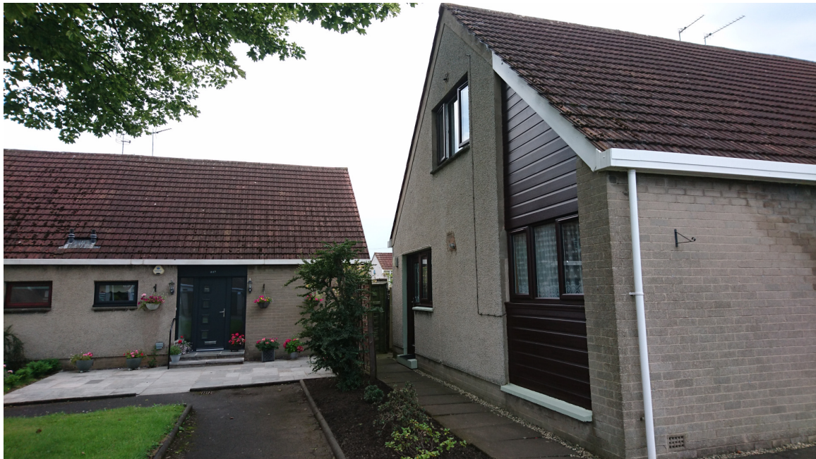
Gable windows looking straight into neighbour front garden.
