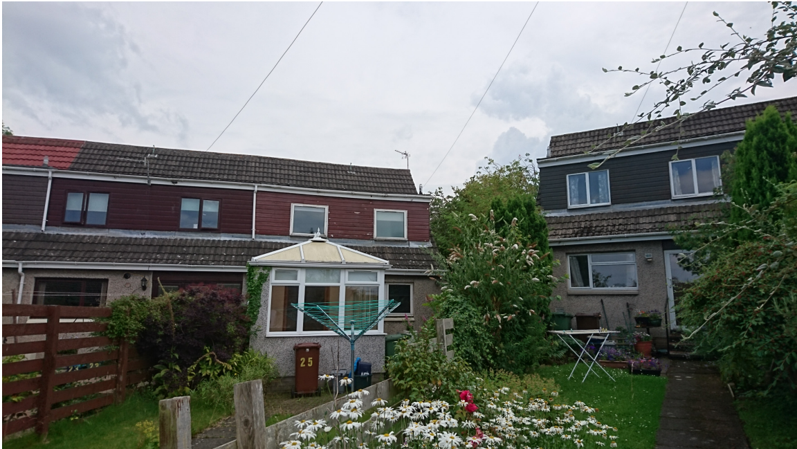
3 separate plots all have dormer windows looking across each other's boundaries.
