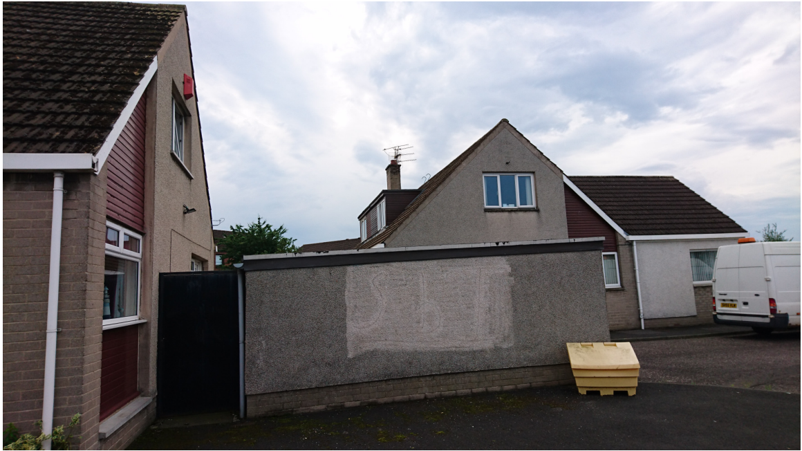
Gable end and dormer windows overlooking neighbour land.
