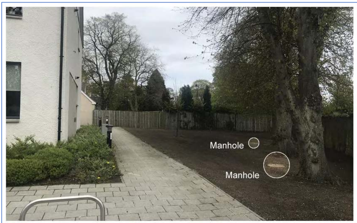
PLATE 18 Victoria Park development showing area of incursion into RPAs for paving, foundations and drainage
