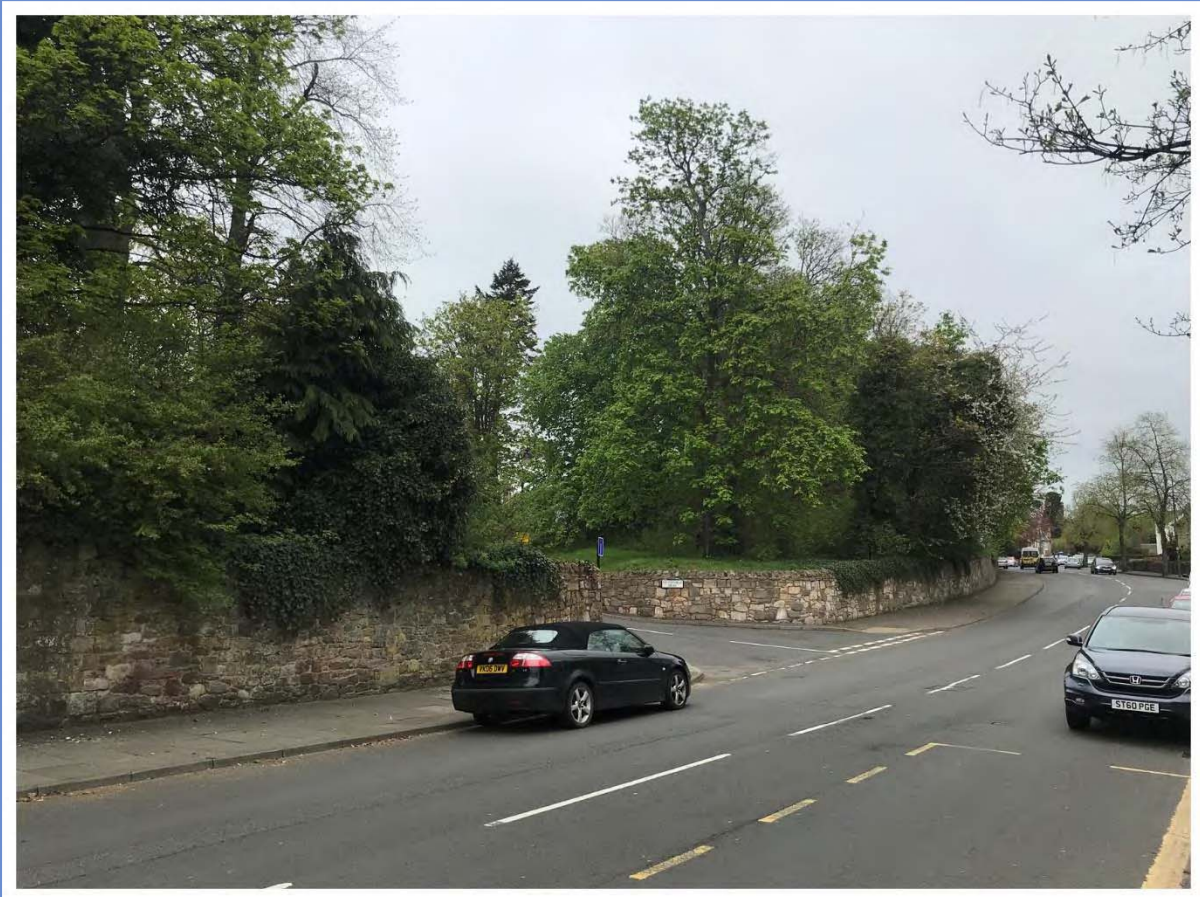
PLATE 7 Application site and Tenterfield House grounds viewed from northern approaches along Dunbar Road
