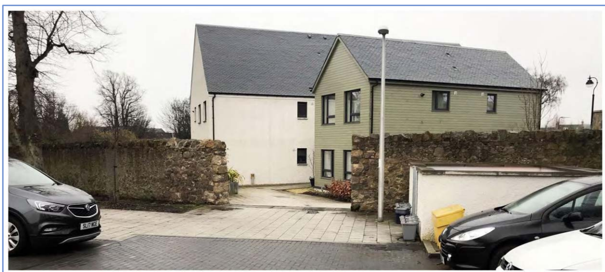
PLATE 3 Old Town Wall as viewed from the Victoria Park development with 4.5m of wall demolished
