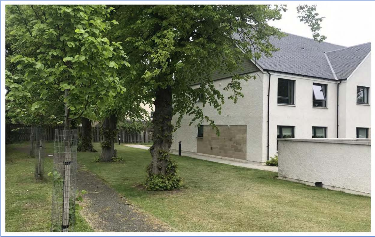
PLATE 17 Victoria Park development showing area of incursion into RPAs for paving and foundations
