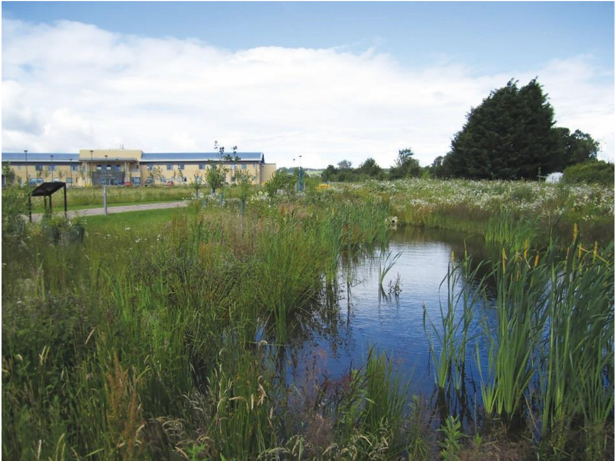
Figure 16: Pond example with barrier planting preventing access to standing water and interpretation board with information on the requirements for and biodiversity value of the pond. Source: The SuDS Manual C753
