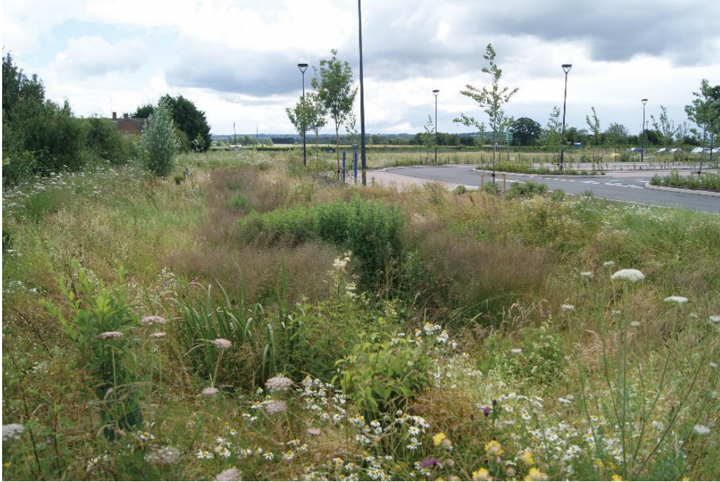
Figure 14: Swale planted for biodiversity and amenity, adding to placemaking principles by being distinctive and welcoming. Source: The SuDS Manual C753
