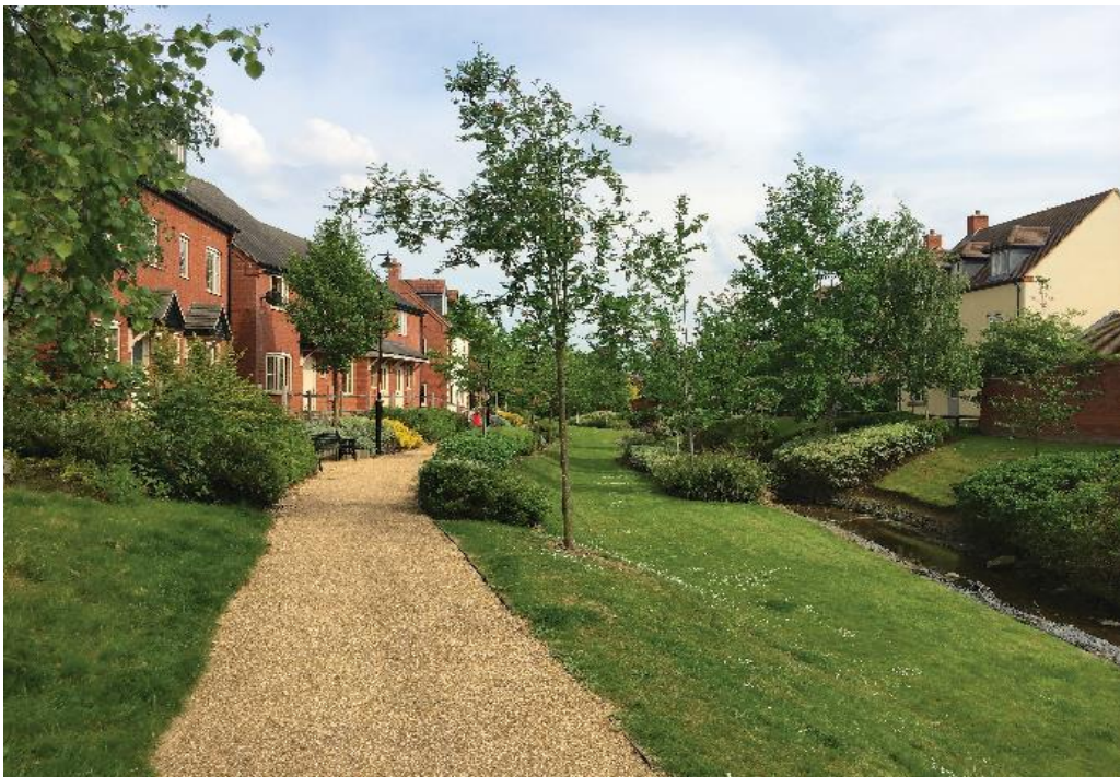
Figure 15: Wet swale example contributing to placemaking by creating attractive and distinctive space that is overlooked to be safe and pleasant, shallow slopes to be easy to move around, and being adaptable and resource efficient. Source: The SuDS Manual C753
