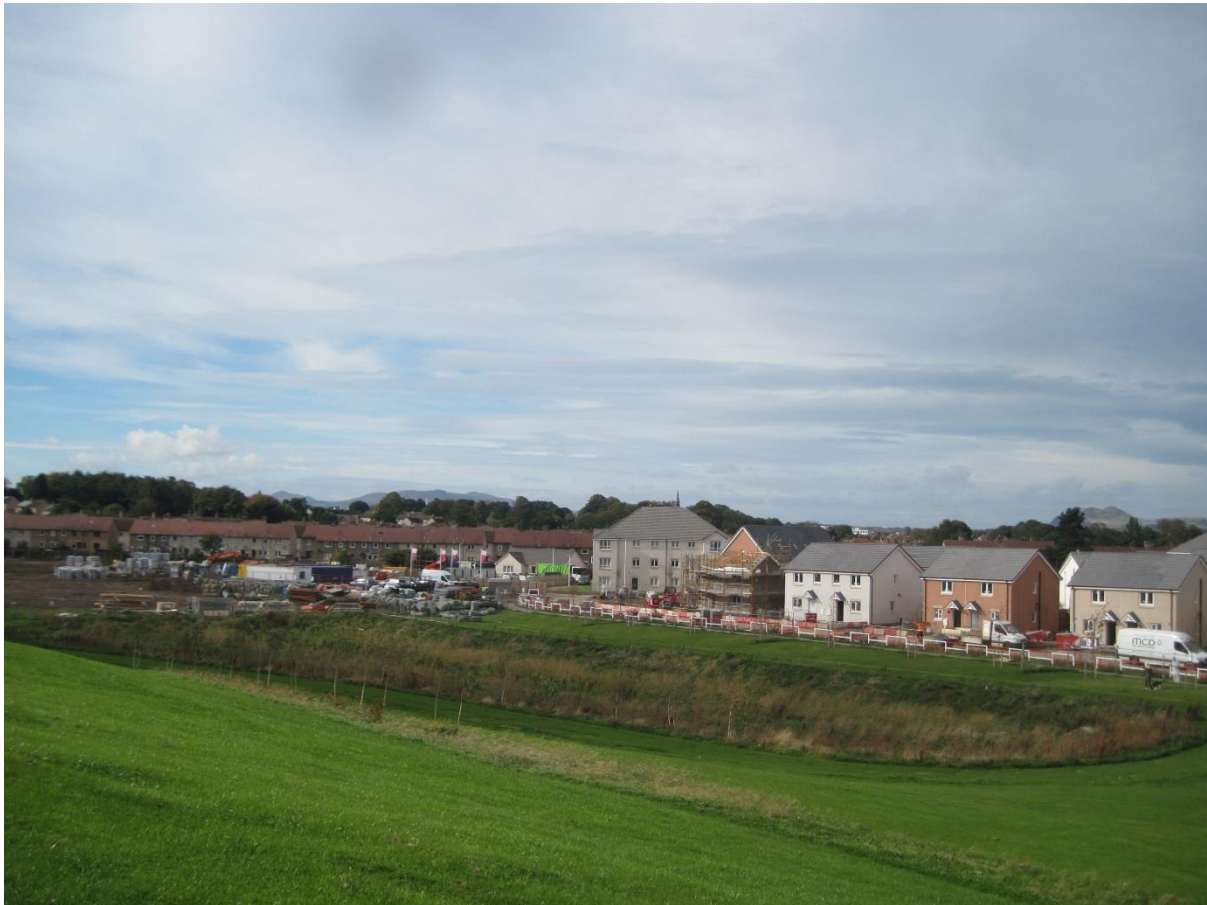
Figure 7: A SuDS basin within a larger area of landscaping creating an attractive landscaped area that is distinctive, welcoming, safe and pleasant, adaptable and resource efficient. Pinkie Park, Battlefield Drive, Musselburgh. Source: author's photo
