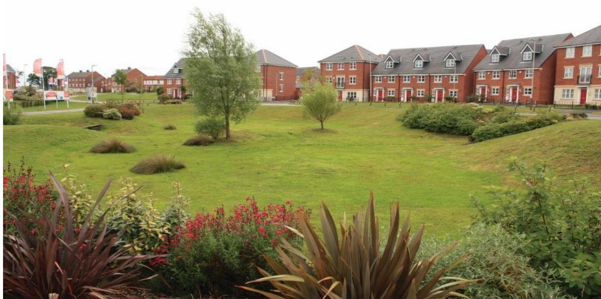
Figure 1: Detention basin providing water detention as well as usable attractive amenity space with a wide base and relatively shallow slopes. Source: The SuDS Manual C753
