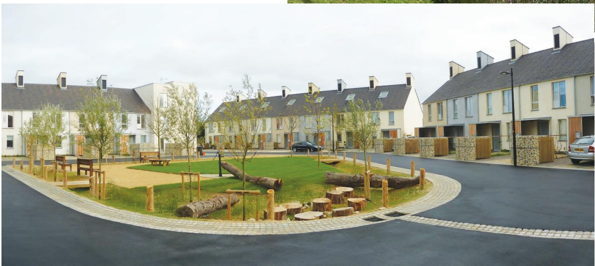
Figure 10: Natural play within a shallow swale providing distinctive adaptable and resource efficient space that is well overlooked and has high amenity value. Source: The SuDS Manual C753
