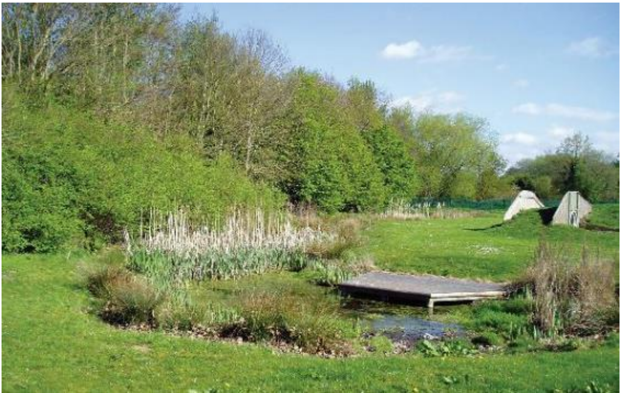
Figure 17: Pond example with dipping platform over shallow water. Source: The SuDS Manual C753
