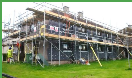
External wall insulation is installed on housing at Pinkie Braes, Musselburgh
