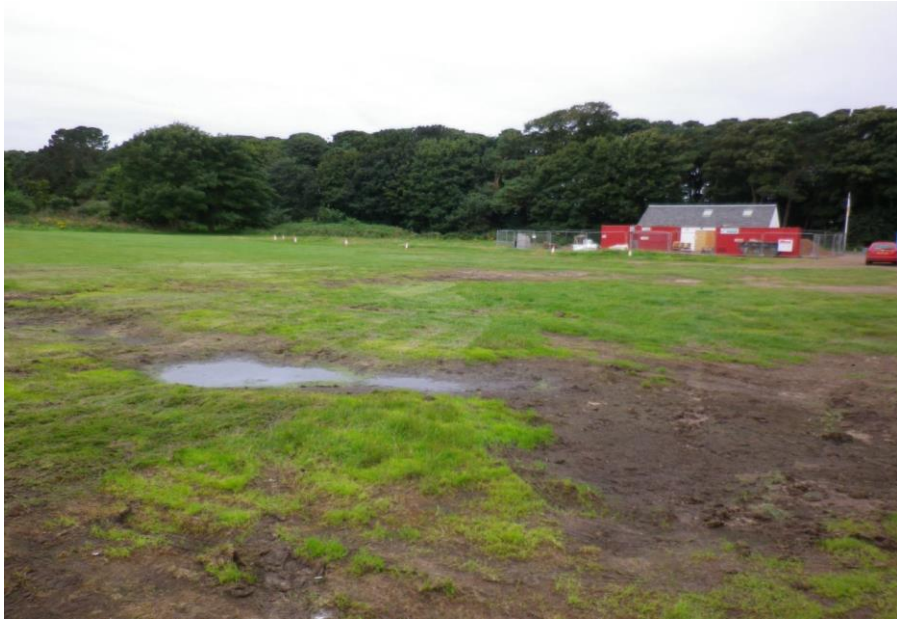
Yellowcraig Car Park Surface
