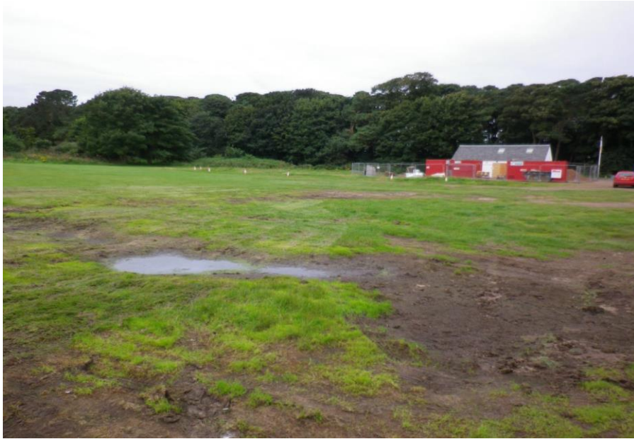
Yellowcraig Car Park Surface
