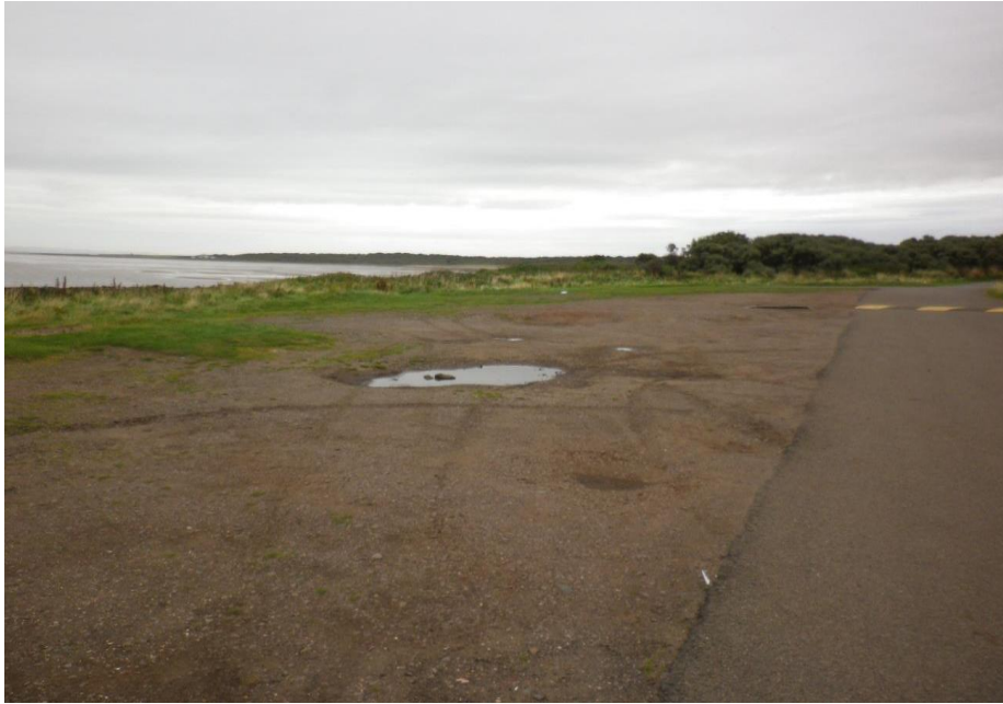
Longniddry No 3 Parking Surface
