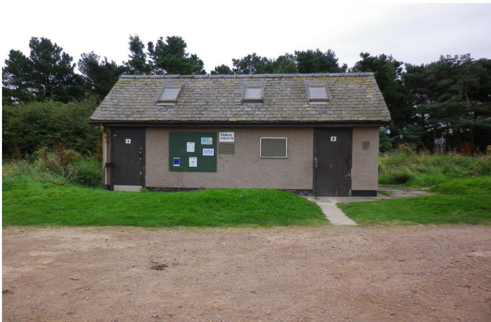
Longniddry No 2 Toilets
