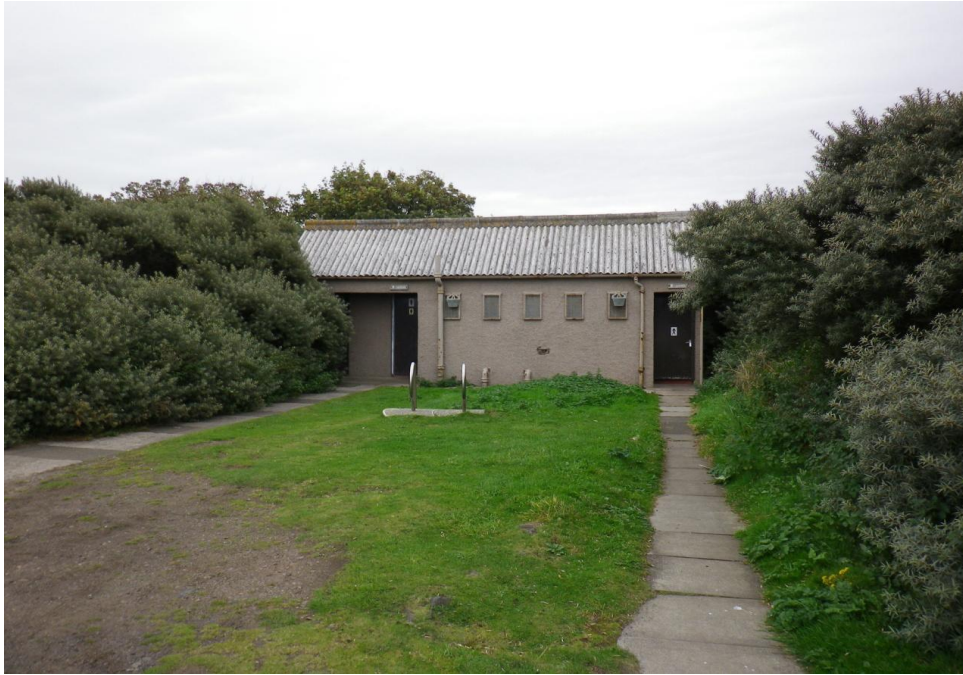
Longniddry No 3 Toilets
