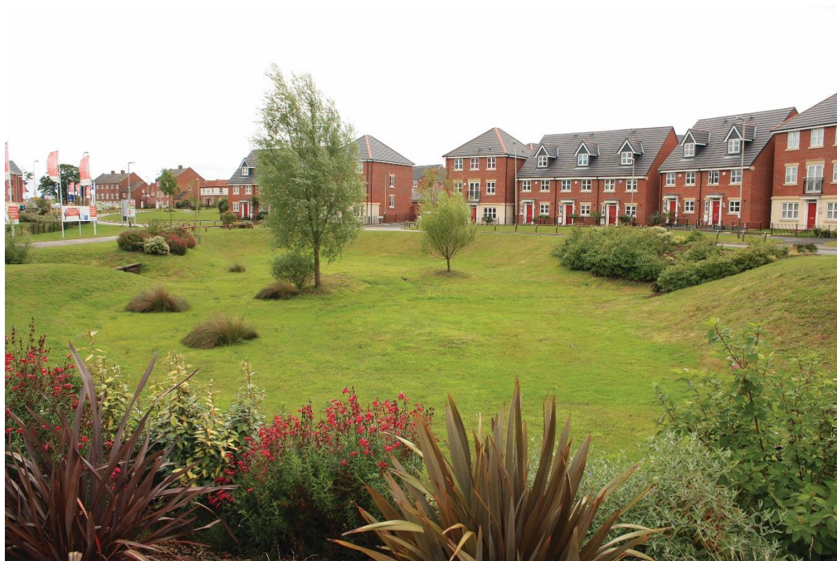
Figure 1: Detention basin providing water detention as well as usable attractive amenity space.
