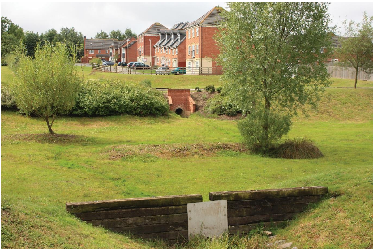
Figure 3: Detention basin providing water detention as well as usable attractive amenity space with raised areas for planting and a variety of side slope gradients. Source: The SuDS Manual C753
