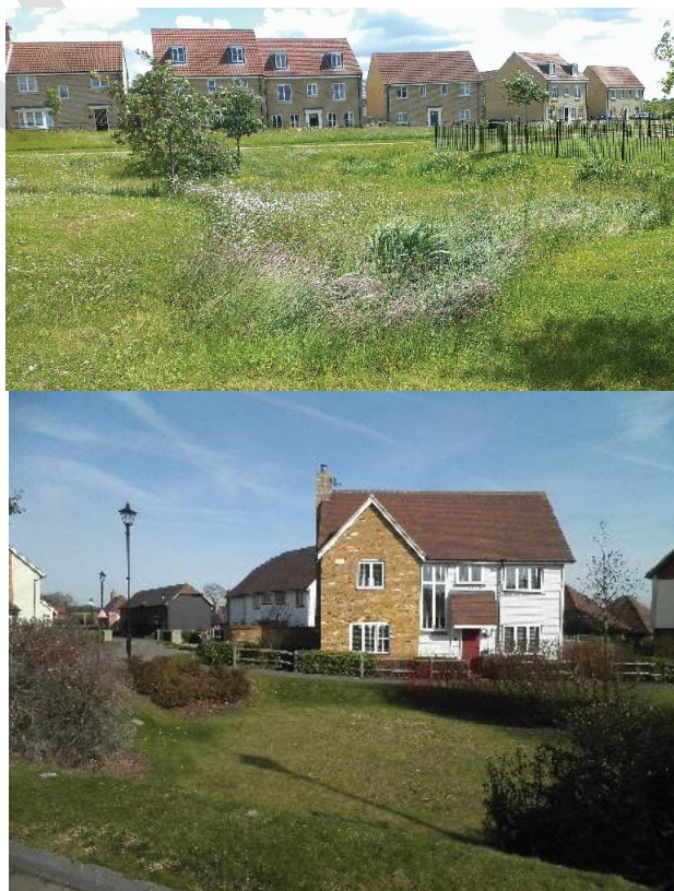
Figure 2: Detention basins with amenity planting and easy access for maintenance
