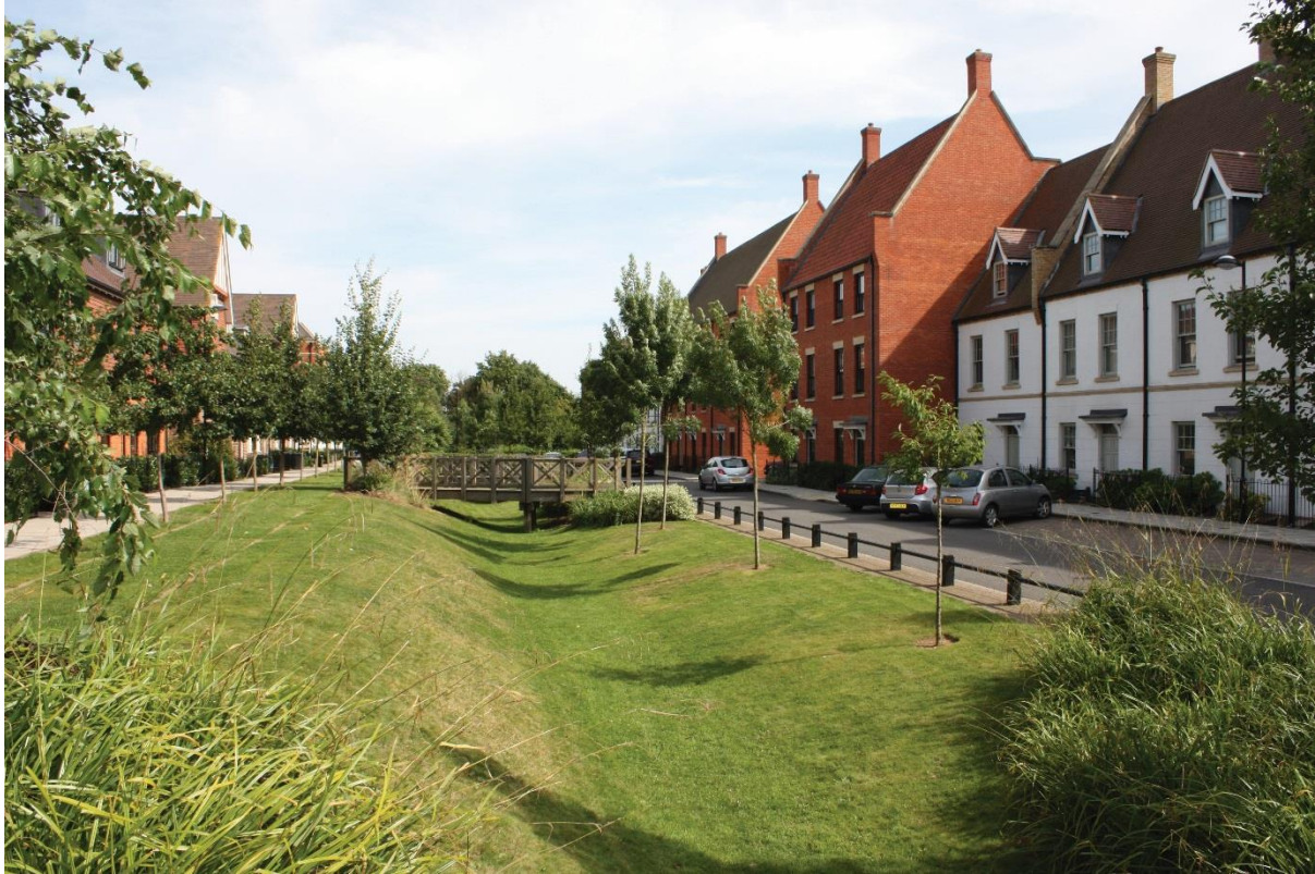
Figure 4: Shallow formal grassed swale wide and shallow enough to be cut by a ride-on mower. Note low fence to prevent vehicle over-run. Source: The SuDS Manual C753
