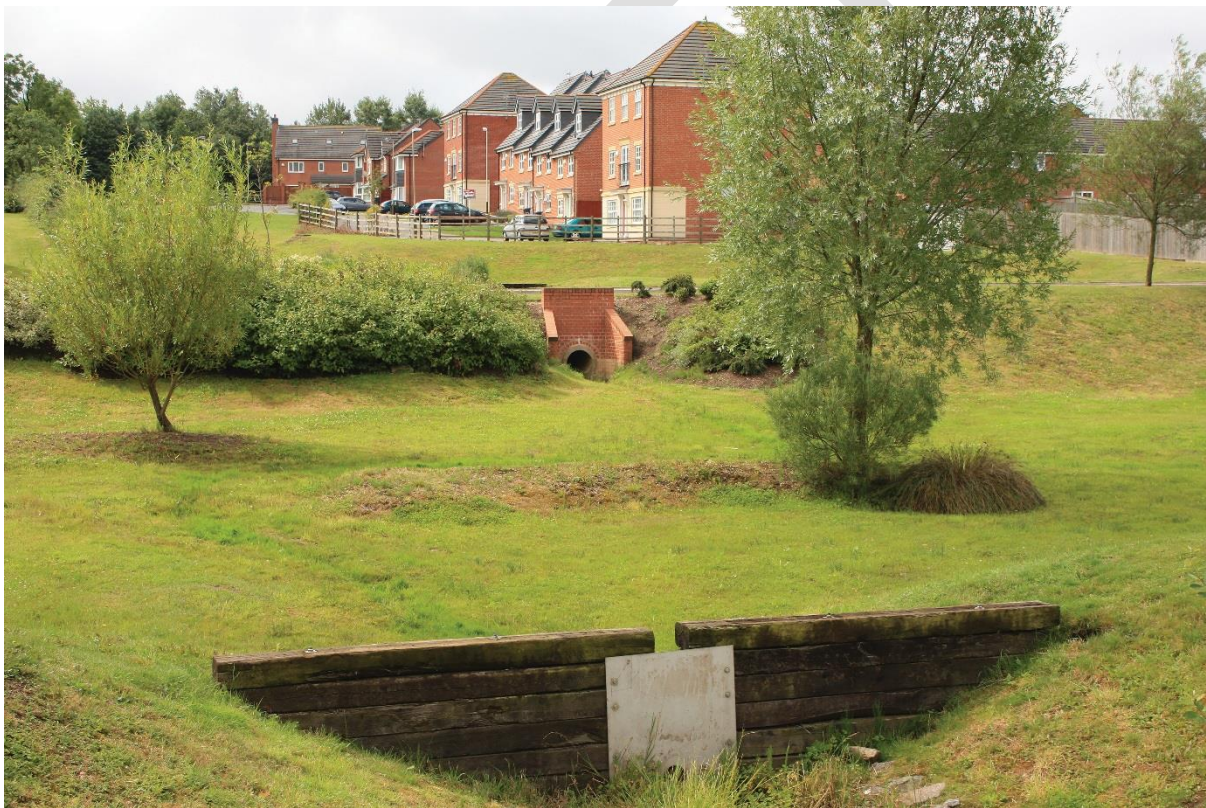
Figure 3: Detention basin providing water detention as well as usable attractive amenity space with raised areas for planting and a variety of side slope gradients. Source: The SuDS Manual C753
