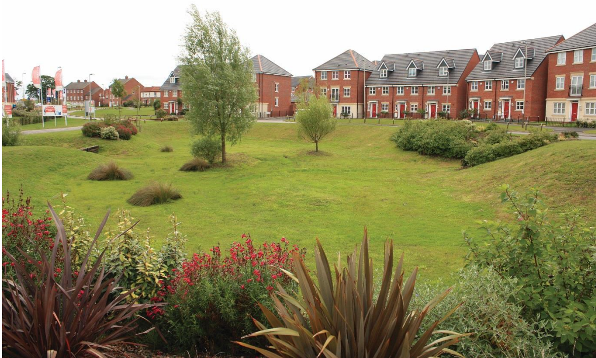
Figure 1: Detention basin providing water detention as well as usable attractive amenity space.
